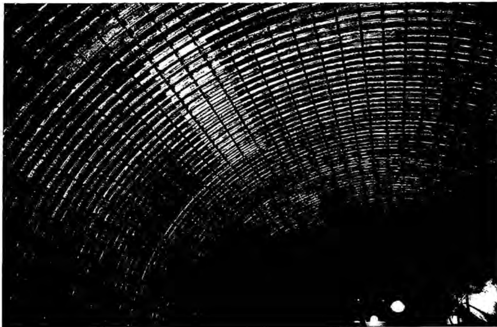
Fig.2-5 Tunnel lining by FRP grids
