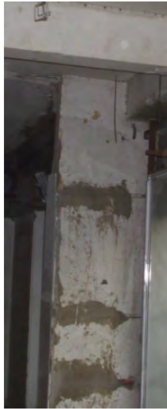
Fig. A-4 Photos of column crack repair.
