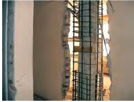
Fig.A-3 Photos of columns Jacketing
