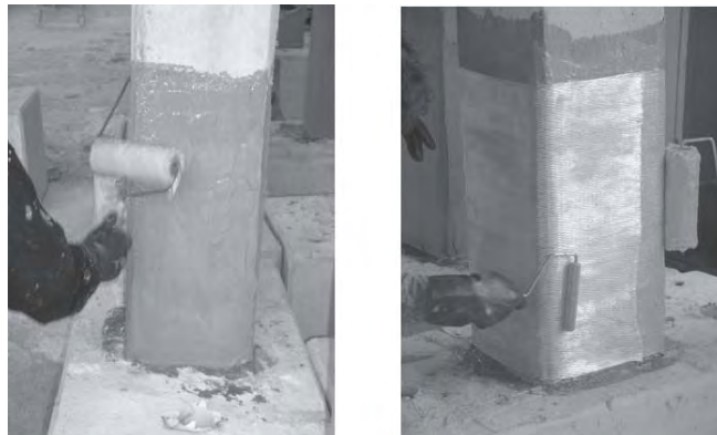
Fig. 5.10 – Wet lay-up confining system.
