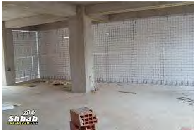
Fig. A-2 Photos of columns before strengthening
