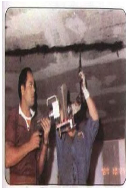
Fig. C-5 Crack injection for slab.
