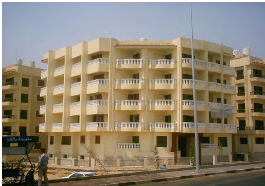
Fig. B-1 view for the building
