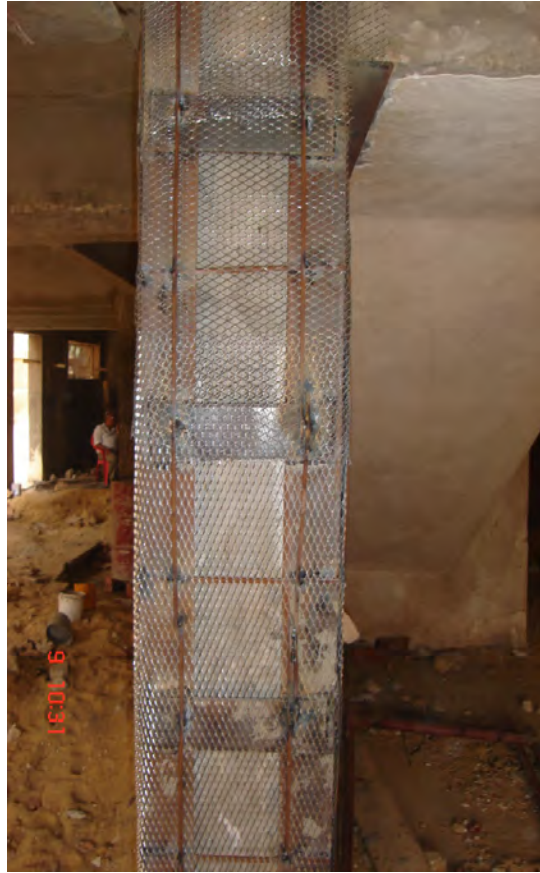
Fig. B-6 column steel jackets.
