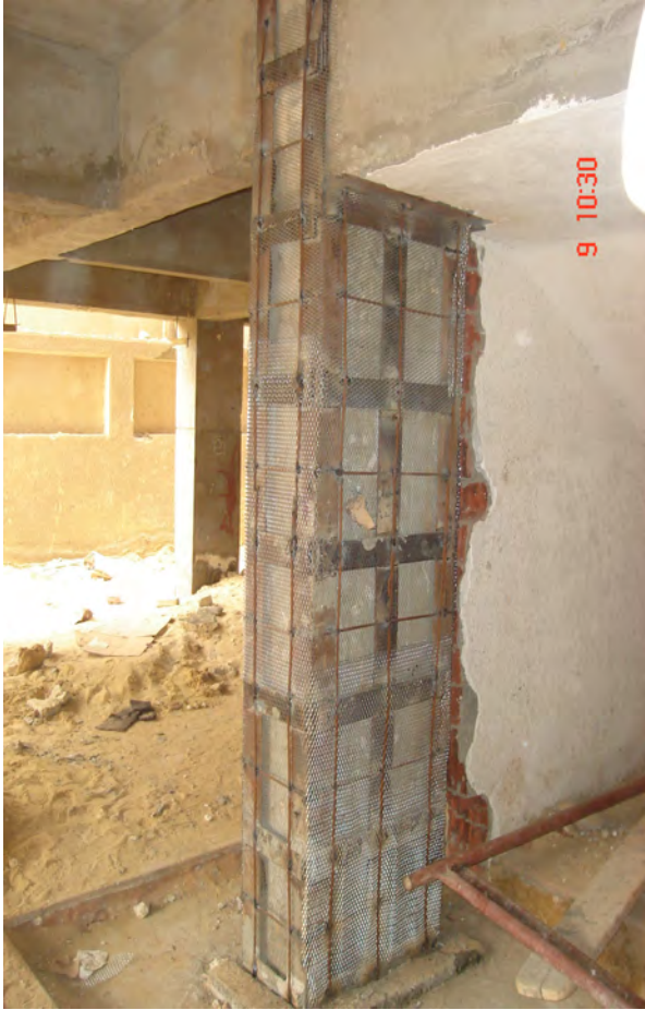
Fig. B-6 column steel jackets.
