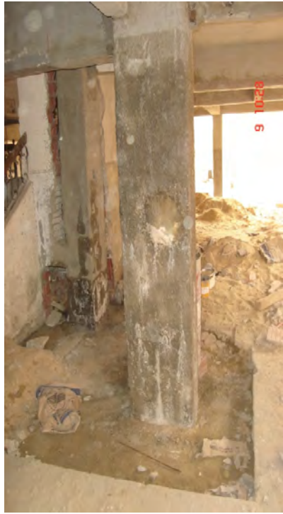
Fig. B-3 Column Photos before strngthening
