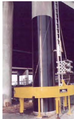
Fig. 5.12 – Automated RC column wrapping.
