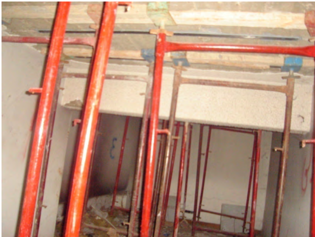
Fig. C-7 Transform load from slab by Steel form
