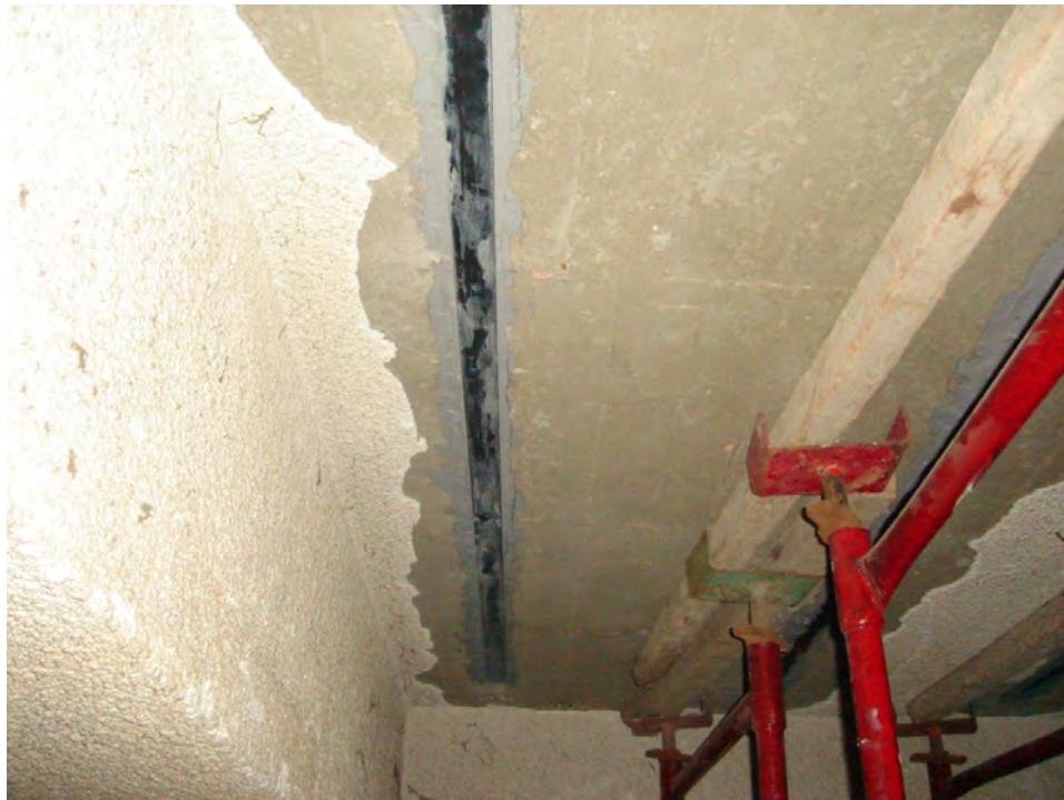
Fig. C-8 Put CFRP to Strength Slab
