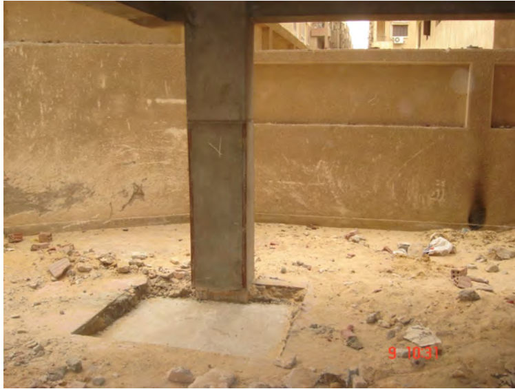
Fig. B- 9 Photos of columns After finish placement of concrete
