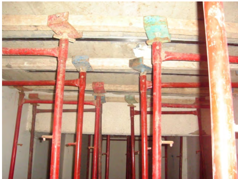
Fig. C- 6 Transform load from slab by Steel form
