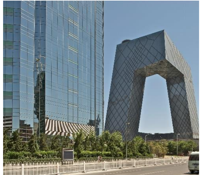
Fig. 10 CCTV Headquarters in Beijing. [15]
