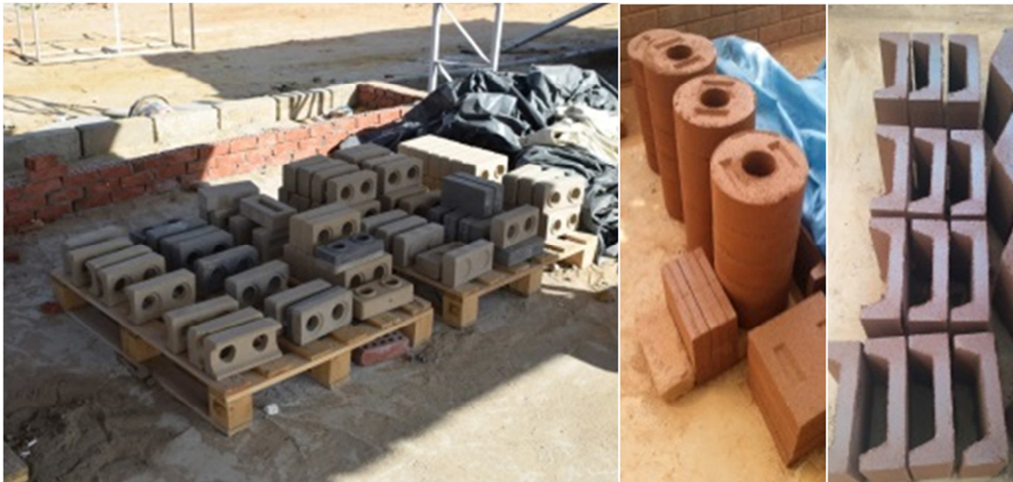
Figure 10. Stacking CSEB units at MSA CoE (left) and AVEI (right).
