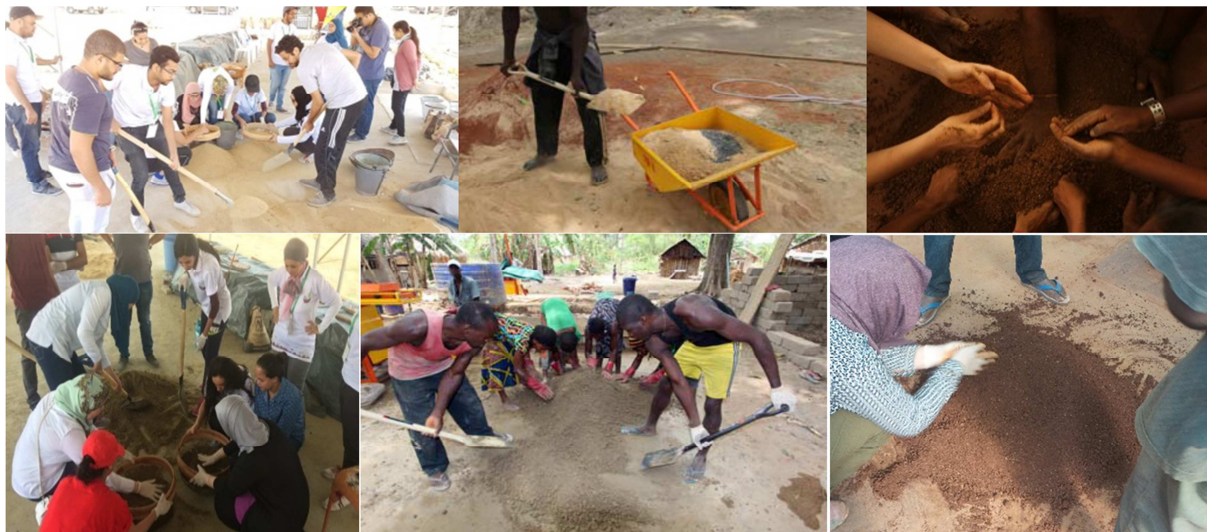
Figure 7. Dry and wet mixing of soil at MSA CoE (left) and AVEI (middle & right).
