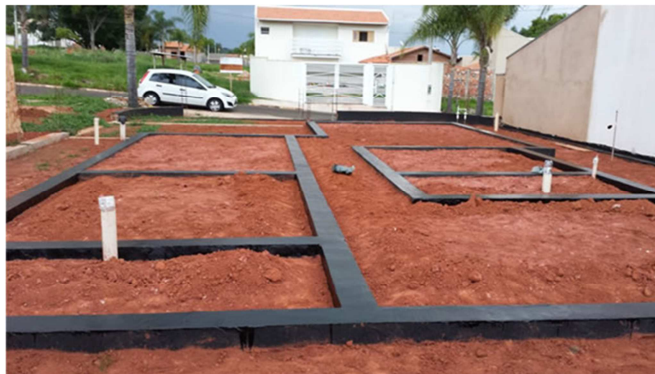
Figure 12. Ground reinforced concrete beams: right, cross section; left, after completion. Source: ecomaquinas.com.br.
