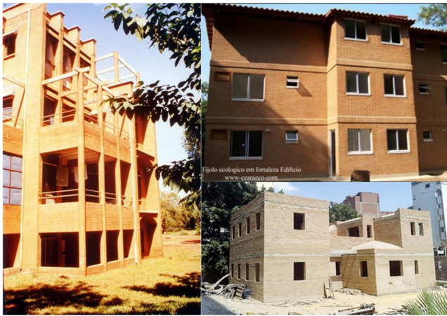
Figure 13. Example buildings showing maximum building heights. Left, India (Vikas community in Auroville); upper right, Brazil (apartment building in Natal RN Brazil); lower right, Egypt (experimental building at HBRC location).
