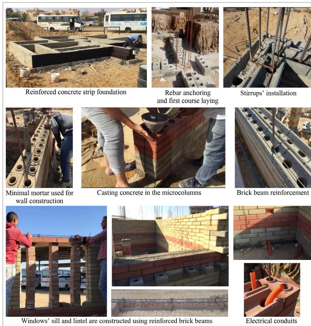
FIGURE 3 Parts of the construction process of EH walls (Source: authors).
