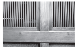
Fig.10. A detail of the removable frame, pillar, and stile. (The author, a survey in Kanazawa City)
