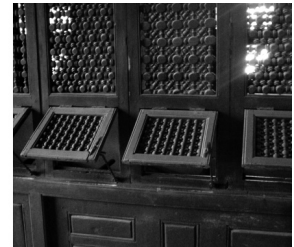
Fig.6. The Keretleya house, mashrabiyya of the harim overlooking the ground floor qa'a . (The University of Liverpool Online Higher Education)
