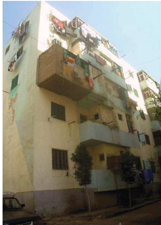
Figure 7: An extended room using wood and bricks in Masaken Zenhom (Source: Author).
