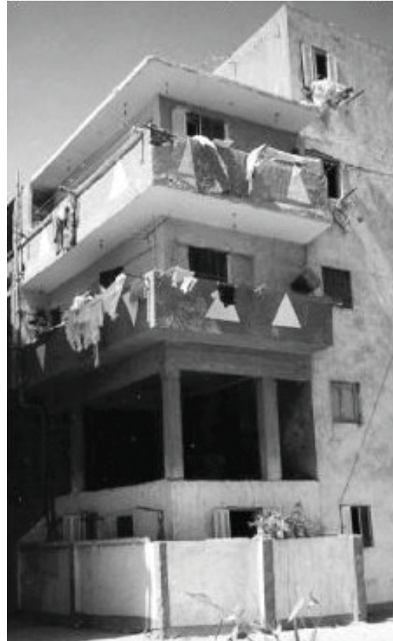
Figure 5: Vertical extensions in an old public housing block in Cairo; the extension provides a large kitchen and a third room (Source: Tipple, 1999).
