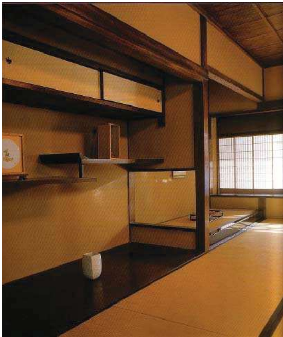
Figure 11: A guest room with a picture alcove (tokonoma) and an ornamental shelving recess (tana) (Source: Black, 2000).
