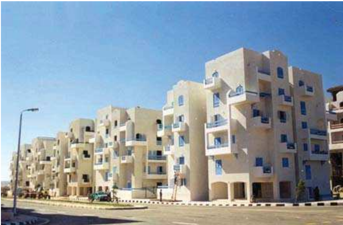
Figure 3: General view of the National Housing Project in 10th of Ramadan City (Source: Arab Contractors official website http://www.arab-contracting.com ).
