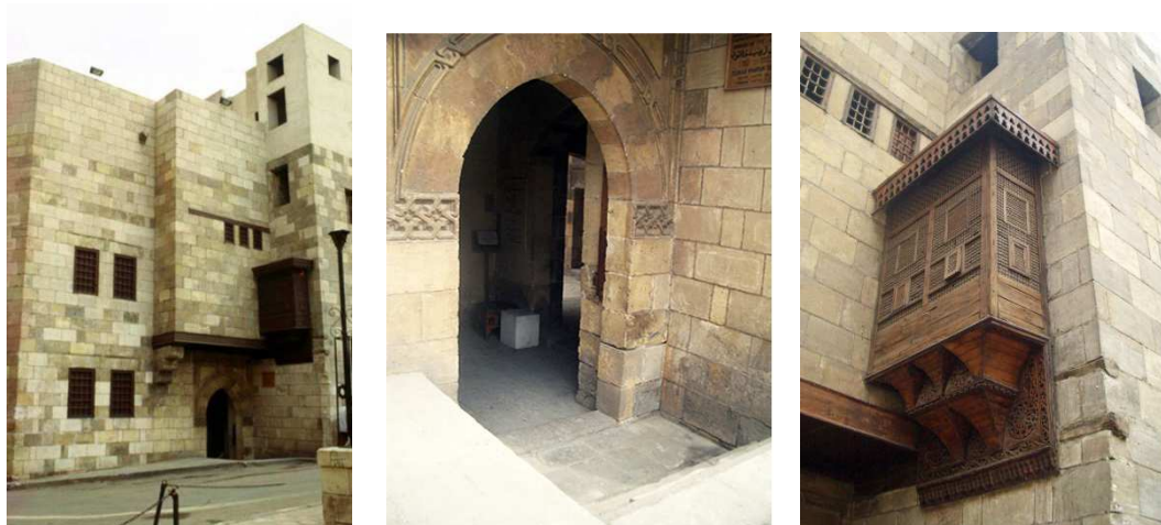
Figure 12: Entrance Façade of Zeinab Khatoun House. Left, general view, source: Aga Khan Trust for Culture, www.archnet.org . Middle, Entrance, source: survey by Abdel Gelil Mohamed, Nermine. Right, mashrabiyya overlooking the entrance, source: survey by Abdel Gelil Mohamed, Nermine.
