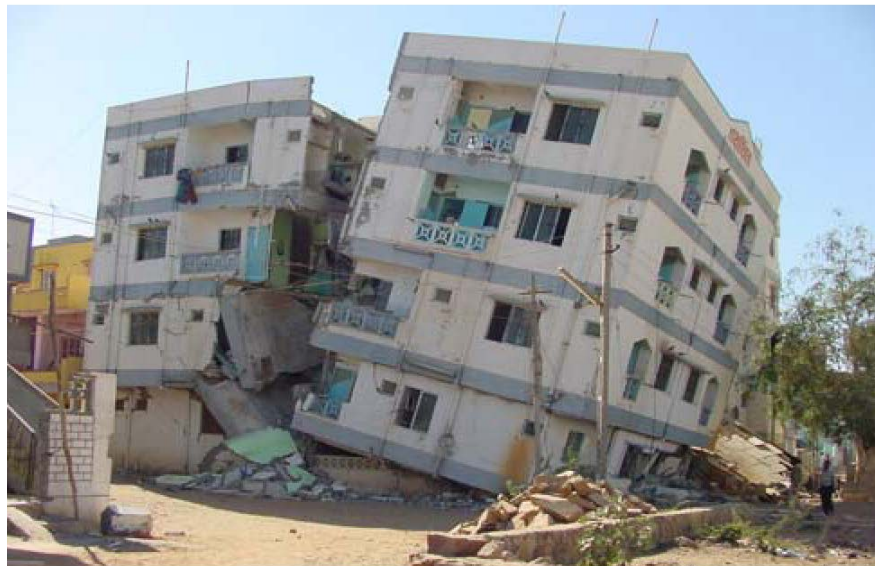
Figure 1.14- Collapse of reinforced concrete columns (and building) during 2001 Bhuj (India) earthquake.
