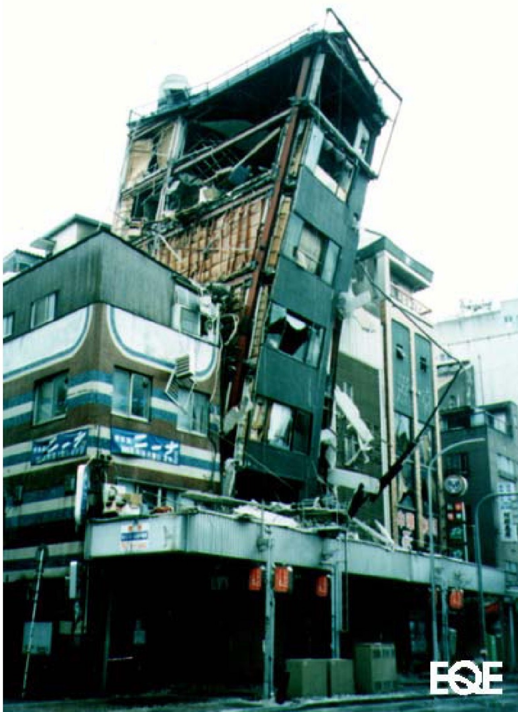
Figure 1.17- Bending of building, Kobe earthquake. (Photo from: The January 17, 1995 Kobe Earthquake.
