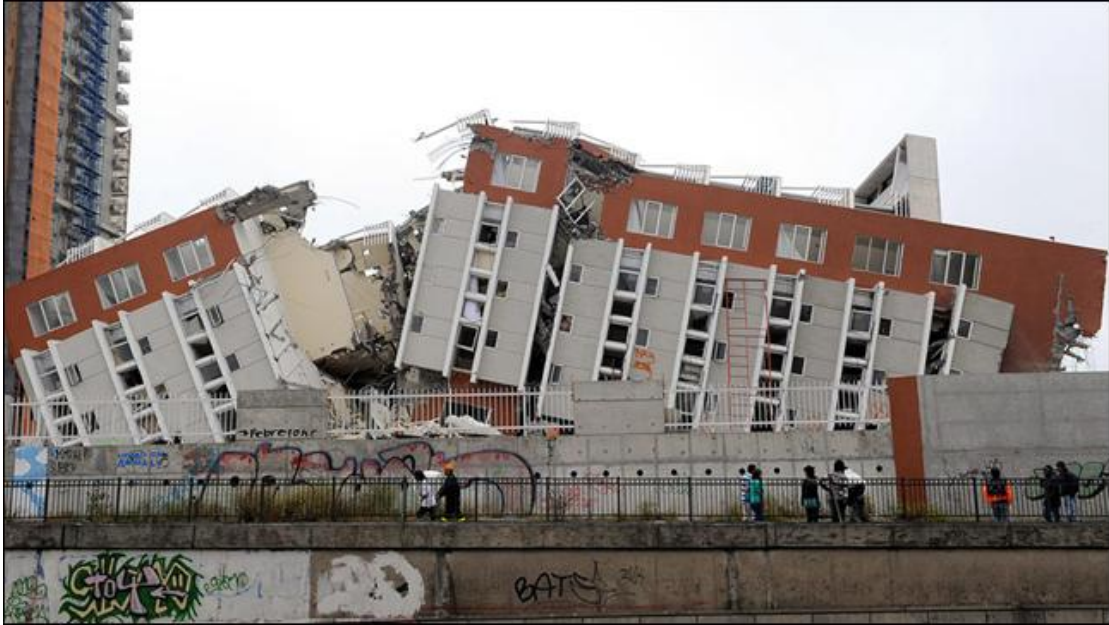
Figure 1.15- Catastrophic earthquake damage to the Alto Rio building, Concepcion, Chile due to the February 27, 2010 M8.8 Earthquake
