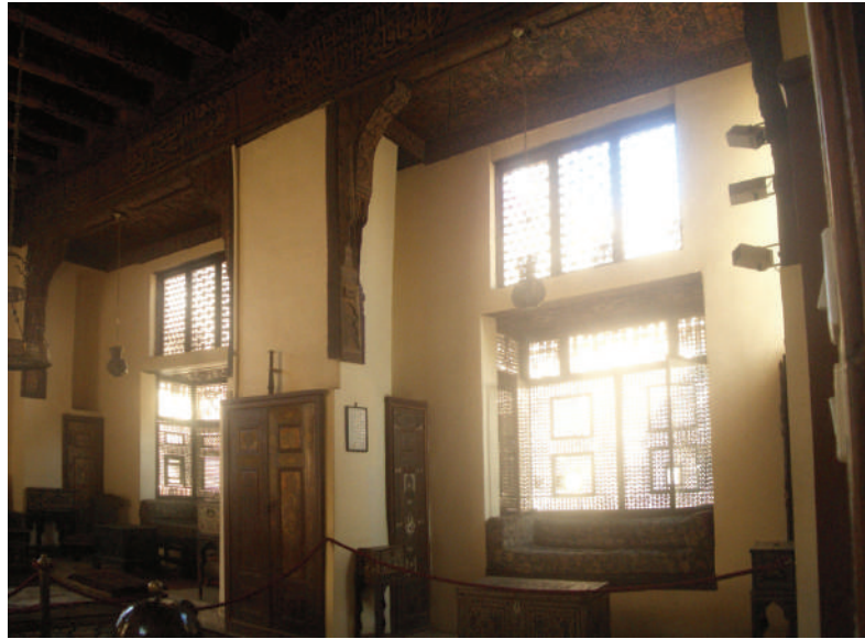
Fig.57. Mashrabiyya in the first floor's qa'a of the haramlik , overlooking the street, Manzil al-Kiridliya . (The author)
