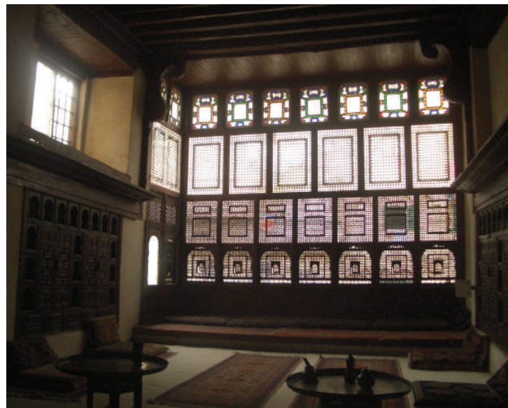
Fig.68. Same mashrabiyya in manzil al-Suhaymi seen from inside (ground floor). The lower tight lattice, upper wide lattice, and the colored glass window in a typical mashrabiyya has been unified to form one large mashrabiyya . (The author)
