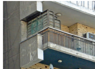
Fig.33. Closing the side of the balcony to protect oneself from the neighbor's eye. Above, an apartment building in Giza; below, an apartment building in Mohandissin, Cairo. (The author)
