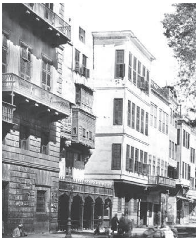
Fig.10. The new balconies and Venetian shutters in a street in Cairo. (In an album dated 1871-2, Egyptian Mirage Collection, the Archive of the Griffith Institute collection, Oxford)
