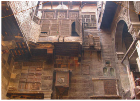
Fig.53. Two Mashrabiyyas in the second floor's qa'a overlooking the Bayt Shabshiri courtyard. (Islamic Art Network)
