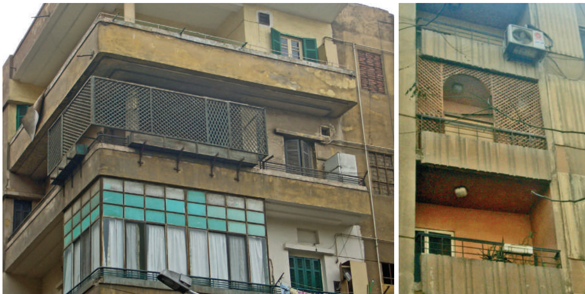
Fig.35. Modifications on the balconies of two apartment buildings. Right, in el-Haram district, left, near Giza Square. (The author)
