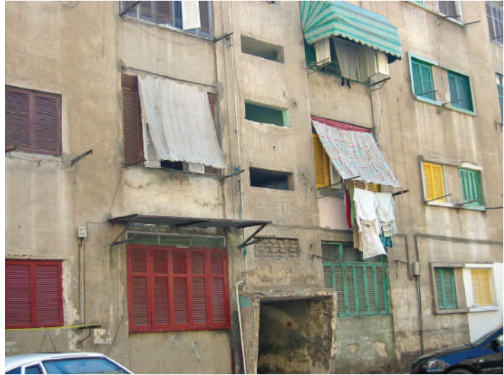
Fig.31. Modifications on a residential building in Imbaba district in Cairo. All these large windows were balconies before people closed it with sheesh . The curtains are fixed to the last washing line to preserve privacy while hanging. Over the washing lines of the ground floor, an overhang is installed, and in the second floor, a shade is installed. (The author)
