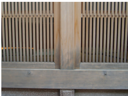
Fig.92. A detail of the removable frame, pillar, and stile. (The author, a survey in Kanazawa city)
