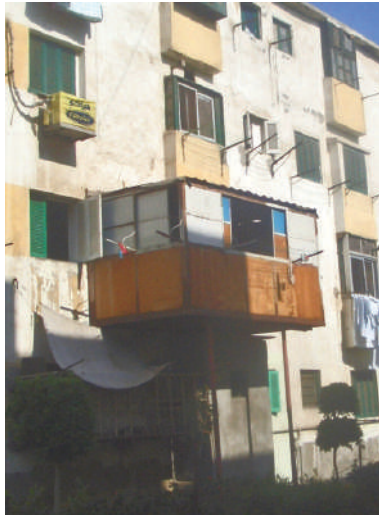
Fig.37. A room added to a unit in Zeinhom Housing. (The author)
