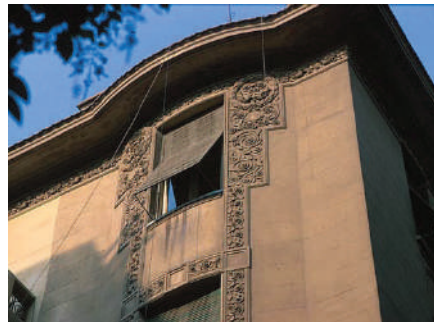
Fig.17. The shutters used during the first half of the 20th century, Garden City. Right, the rolling shutter opening upward, left, the Venetian shutter divided into two parts. (Photo by Donat Agosti)
