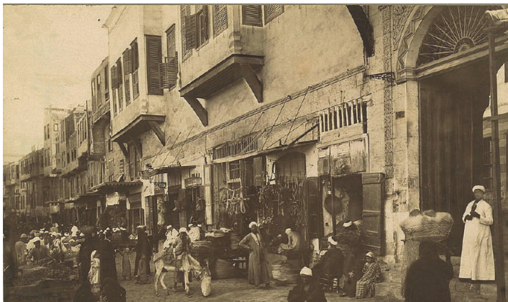
Fig.11. Commercial street in Cairo showing the new upper floors' solid projections with the Venetian shutter divided into two parts. (Photo by Bonfils, between 1867 and 1899, Prints and Photographs Online Catalogue, Library of Congress)
