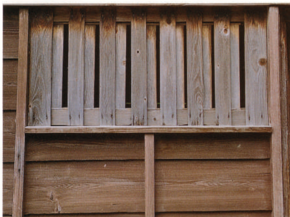
Fig.99. Musō-mado . Left, on a house in Matsue city, Shimane pref. (Ikeda, 1997, p. 46) Right, plan and elevation. (Aoki et al. 1993, p. 1622)
