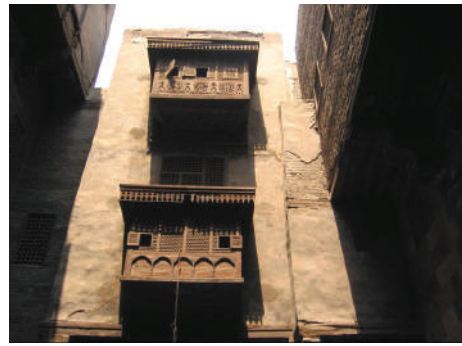
Fig.54. Mashrabiyyas of the haramlik 's main rooms in second and third floor overlooking the Bayt Shabshiri courtyard. (Islamic Art Network)
