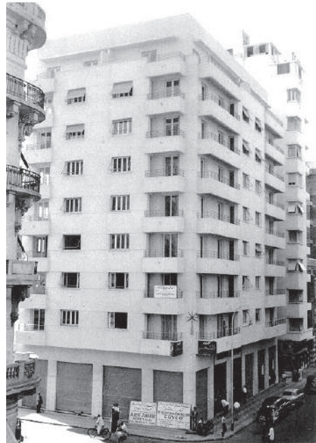
Fig.18. Lababidi apartment building, 1940s, by arch. Albert Zanairi. Modernism identically treated the threshold between the interior and the exterior with open balconies and large windows with glass panels and shutters. (Raafat 1998)
