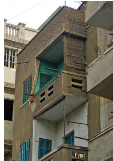
Fig.31. Modifications on a residential building in Imbaba district in Cairo. All these large windows were balconies before people closed it with sheesh . The curtains are fixed to the last washing line to preserve privacy while hanging. Over the washing lines of the ground floor, an overhang is installed, and in the second floor, a shade is installed. (The author)
