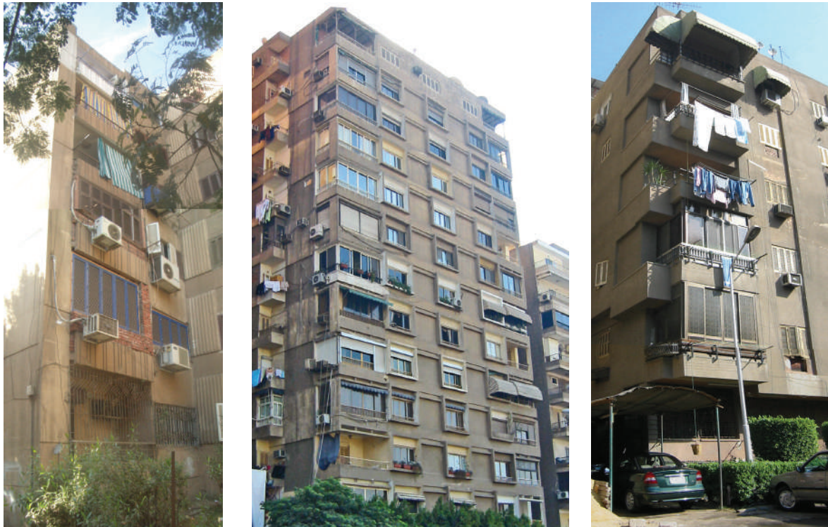
Fig.34. Modifications on the balconies and windows of three apartment buildings in middle and upper class districts in Cairo. Right, el-Sahafiyin (Journalists) district, middle, el-Mohandissin (Engineers) district, and left, el-Haram district. (The author)
