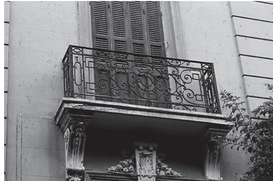
Fig.16. An art nouveau style balcony with a Venetian shutter in Garden City. (Photo by Donat Agosti)
