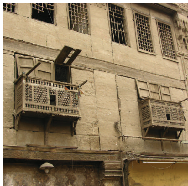
Fig.64. Arrangement and form of the openings of Rab' Qayt-Bay . (ArtServe, the Australian National University)
