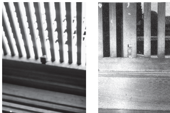
Fig.93. The removable pins of the hamekomigōshi . (Left: the author,; right: Hiyuga 1988, p. 102)
