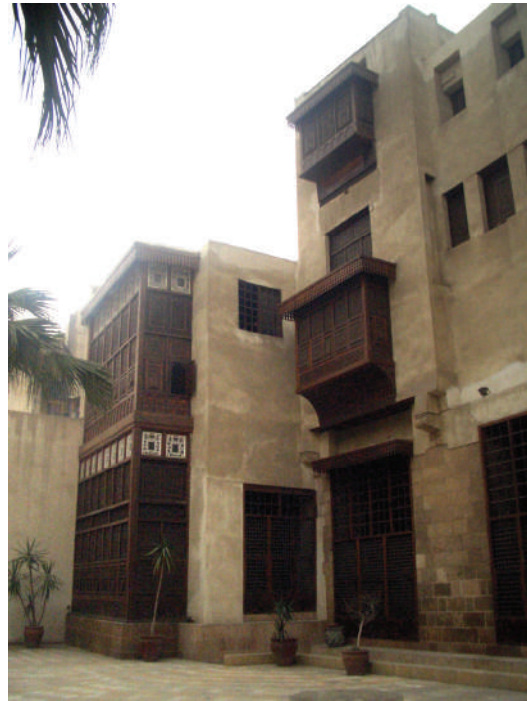
Fig.67. Mashrabiyya covering the entire façade of two qa'as overlooking the northern garden in manzil al-Suhaymi . (The author)
