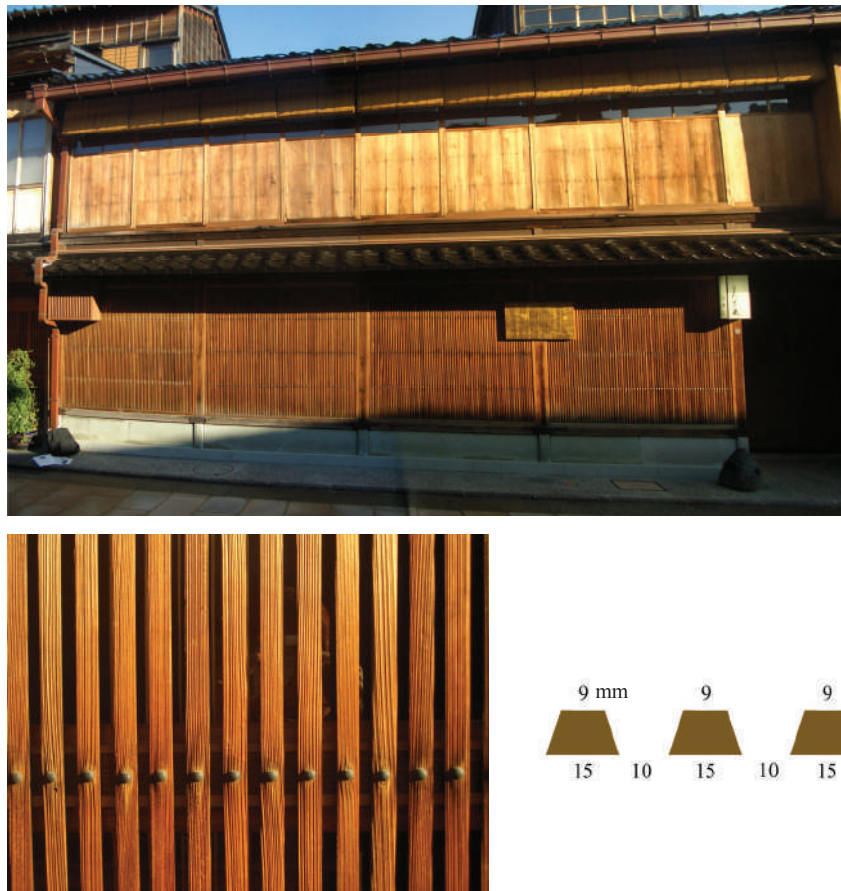
Fig.103. A chaya in Higashi Chayamachi, a former entertainment district in Kanazawa city. Above, façade; below, sasame-gōshi seen from outside and detail of the mullions' cross-section. (The author)
