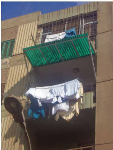
Fig.39. Overhang and shades installed on balconies in Montasser housing, el-Haram. (The author)
