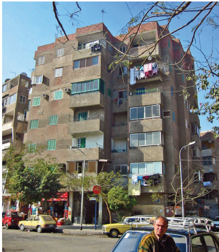
Fig.4. A typical apartment building in Cairo, el-Sahafiyin district.
