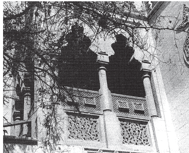
b) Detail of a villa showing the mashrabiyya typically applied over the balustrade. (Asfour 1993, p. 136)
