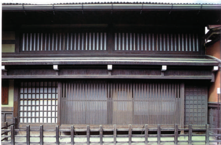
Fig.108. Fukiyose kiriko-gōshi seen from outside and inside. Yoshijima house in Takayama city. (Ando 1997, p. 100)
