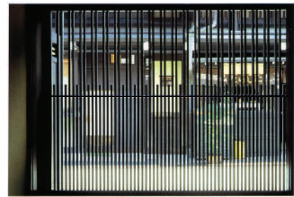
Fig.108. Fukiyose kiriko-gōshi seen from outside and inside. Yoshijima house in Takayama city. (Ando 1997, p. 100)
