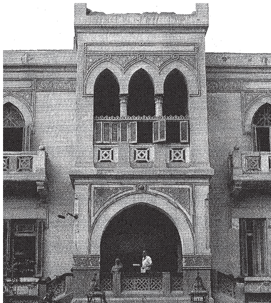
a) Facade of villa of Delbrun Shukri in Hilmiyya with Venetian shutters over the balustrade. (Asfour 1993, p. 135)
