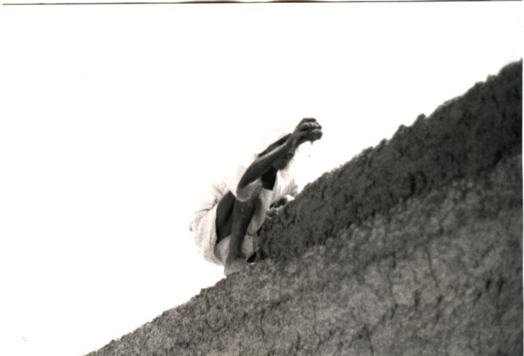
Figure 3.9: Building a House in the Self-Help Quarter.
