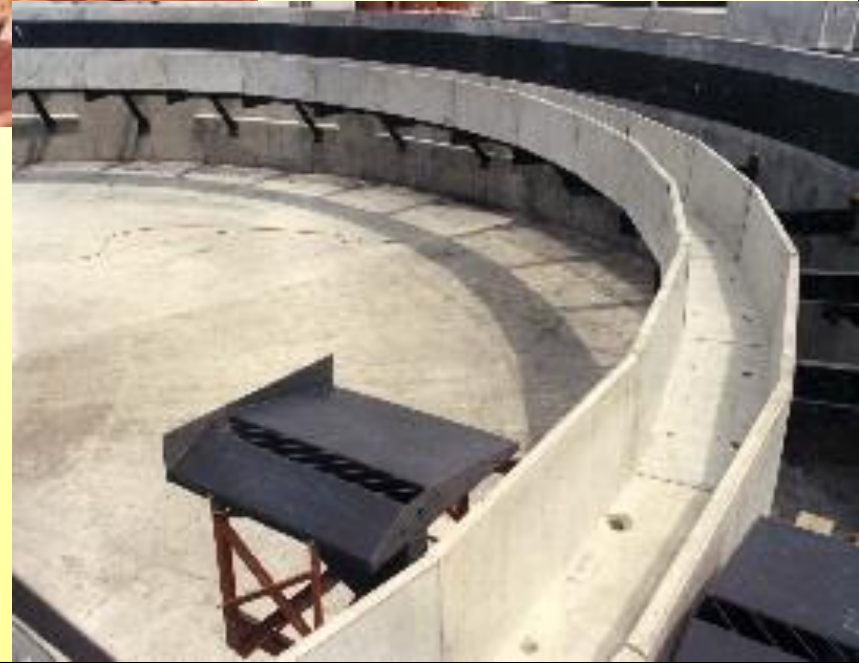
Secondary Clarifier Under Construction
