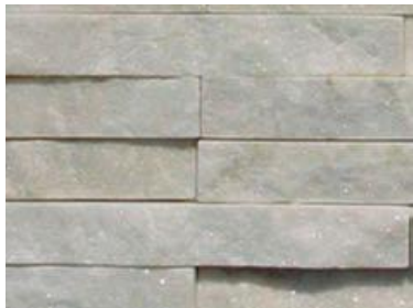
Stone Wall Cladding
