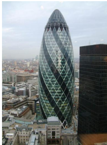
Fig. 1-17 Swiss Re, expressing the use of exoskeleton frame braces and glass.
