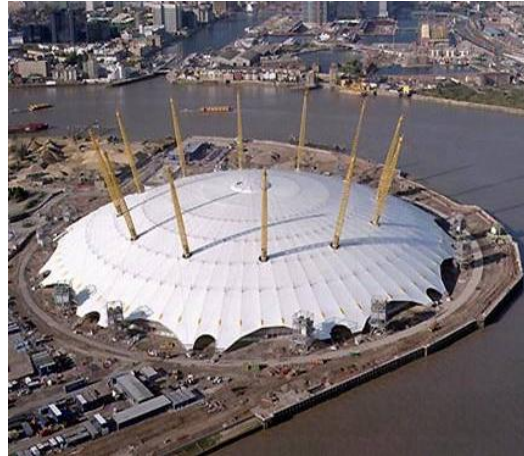
Fig. 1-20 The O2 Arena, expressing the use of PTFE plastic roof.
