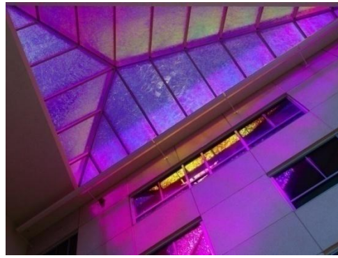
Fig. 3-21 Using dichroic glass in skylight
