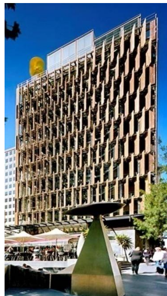
Fig. 4-25 The building when the solar shadings are opened
