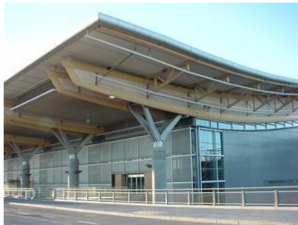
Fig. 1-8 Oslo Airport, expressing the use of timber in the roof structure.
