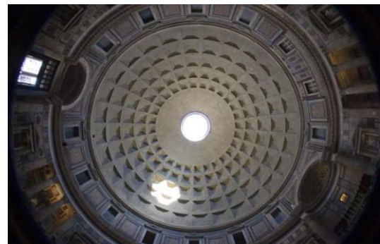
Fig. 1-11 Pantheon, expressing the largest unreinforced dome in the history of architecture.
