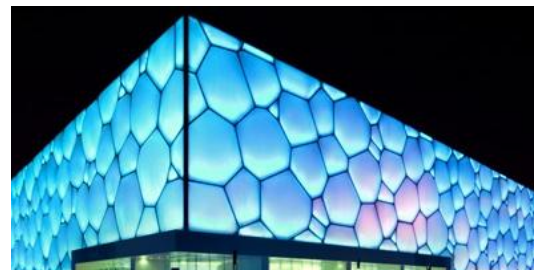
Fig. 1-22 Wter Cube, expressing the clad with ETFE plastic
