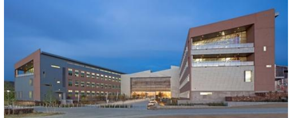
Fig. 4-29 The RSF has a skewed-H-shaped plan defining exterior courtyards. The building's two wings are elongated on the east-west axis to make the most of sunlight for interior illumination.
