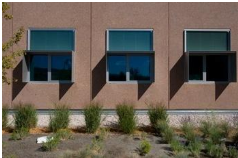
Fig. 4-32 South-facing windows with shading projections surrounding the vision area.
