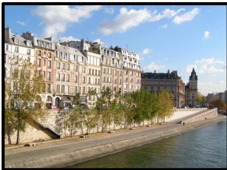
Fig. 4-97 variety and diversity in Ile de la Cité district
