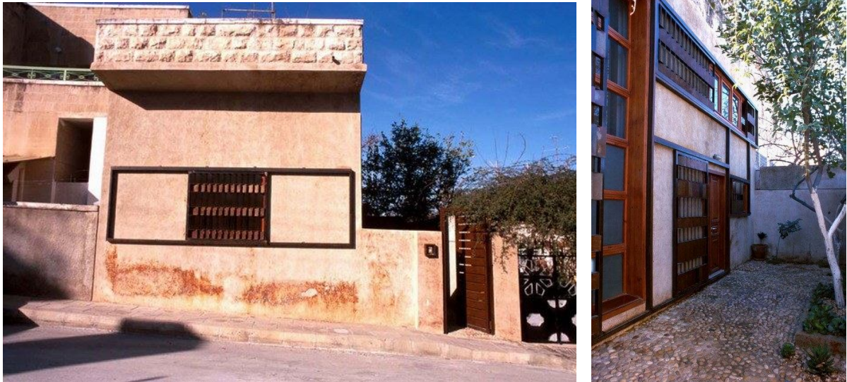
Figure 2.24: Facades with a roughly textured layer of concrete mixed with steel powder. Source: CSBE, 2002.
