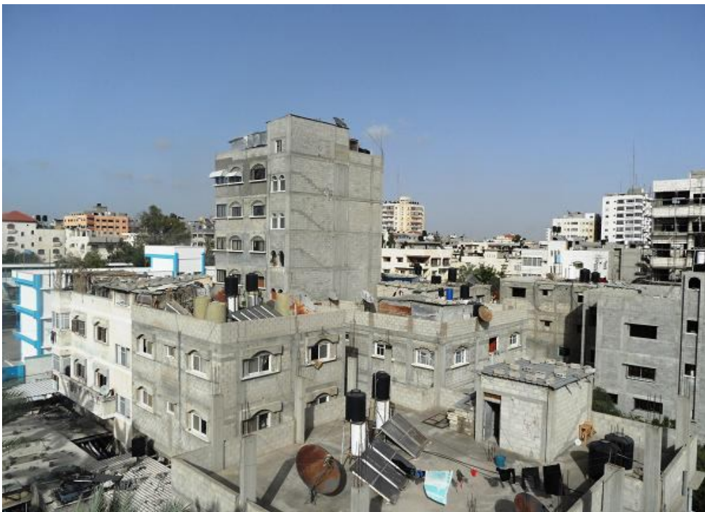
Figure 3.10: Repetitive use of building products and components in the Gaza Strip.
