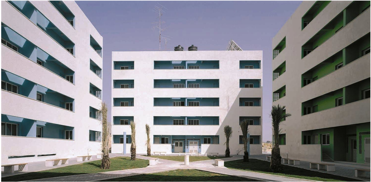
Figure 3.14: External view. Source: Fiedler, 1999.
