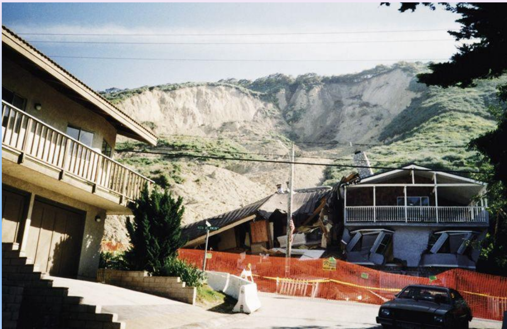
Complex landslide at La Conchita, California (1995)
