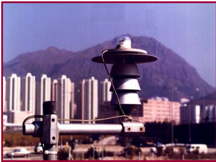
Solar radiation detector
