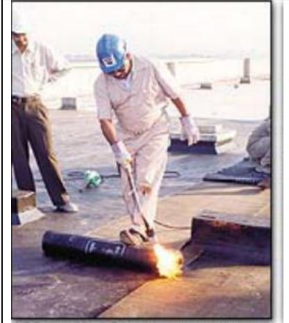
APP modified Bituminous membrane being torch applied.
