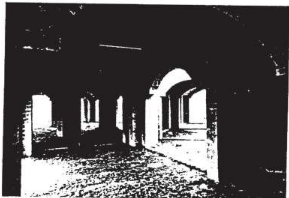
ARCHED AND CORBELLED OPENINGS
