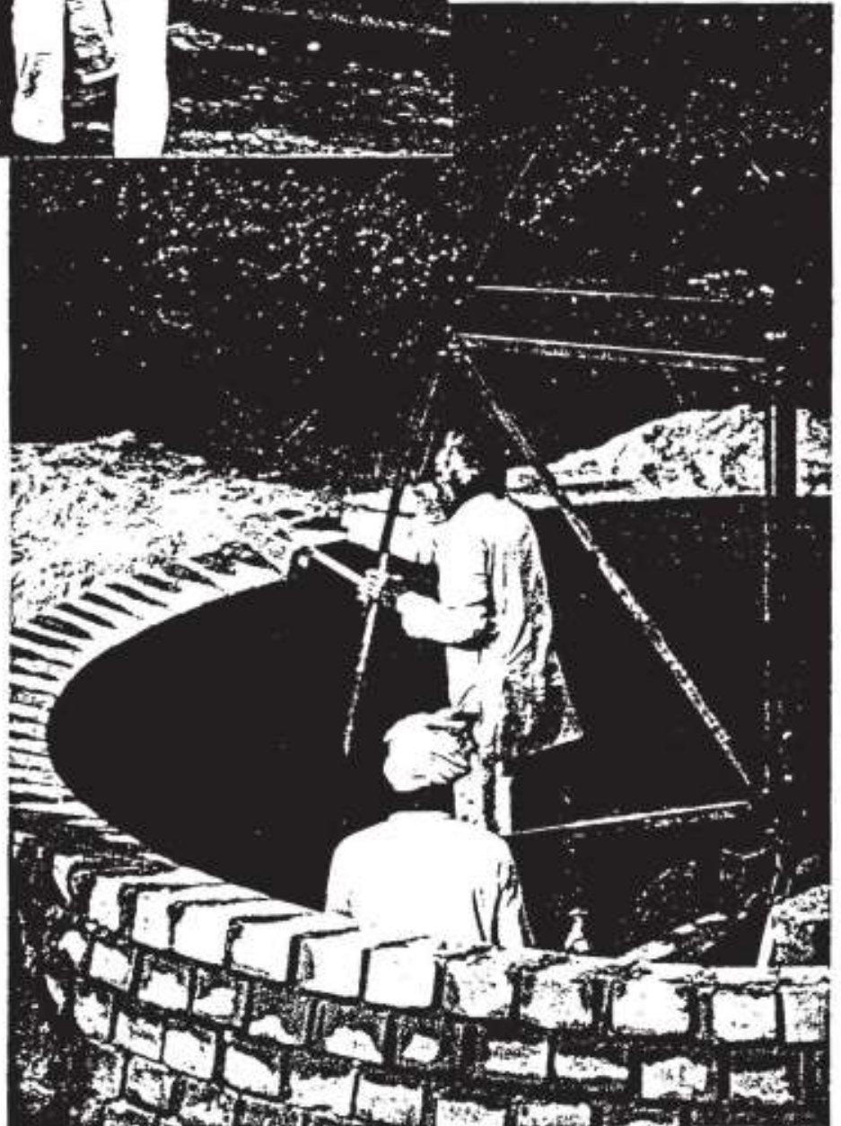
Fig. 3: Construction of a dome with a rotational slip form
