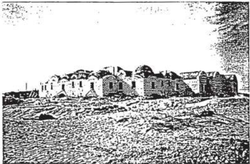
Fig .1 View of DAL building
