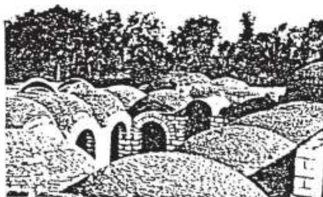
Fig .4 View of domes and vaults construction
