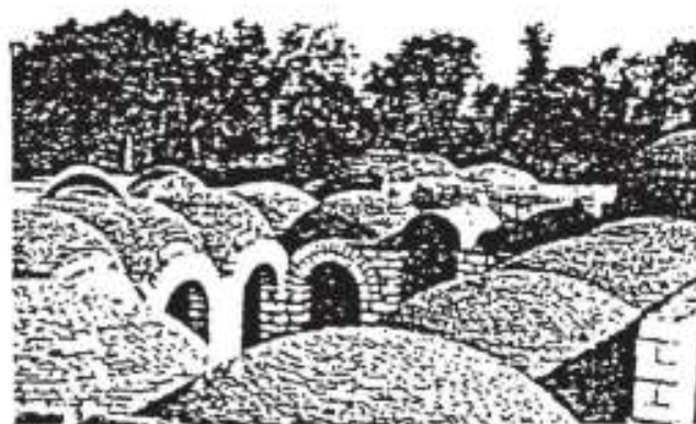
Fig .4 View of domes and vaults construction
