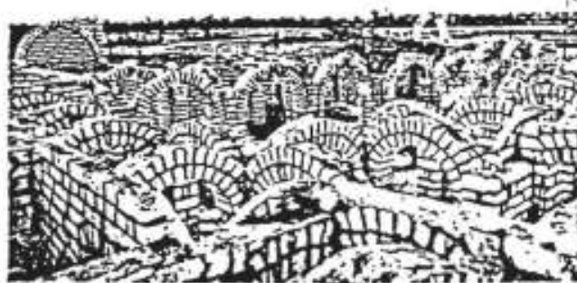
Fig .3 View of bearing walls and arches
