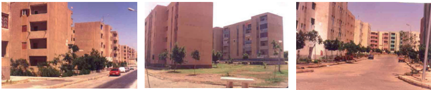
Figure 1: External features of the five story walk-ups.
