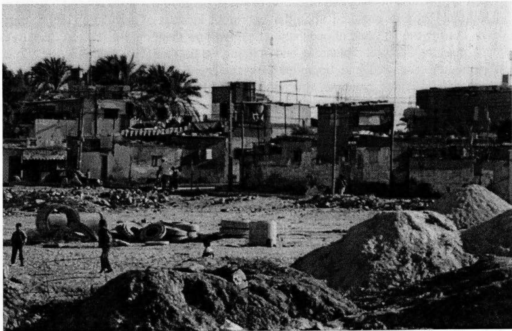
Photo 21: Quarter Renovation in Deir al Balah ( Waltz 1998 )
