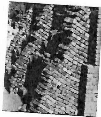
fig.13, the way to keep blocks together safe in a dynamic environment is to have them on an inclined planes.
