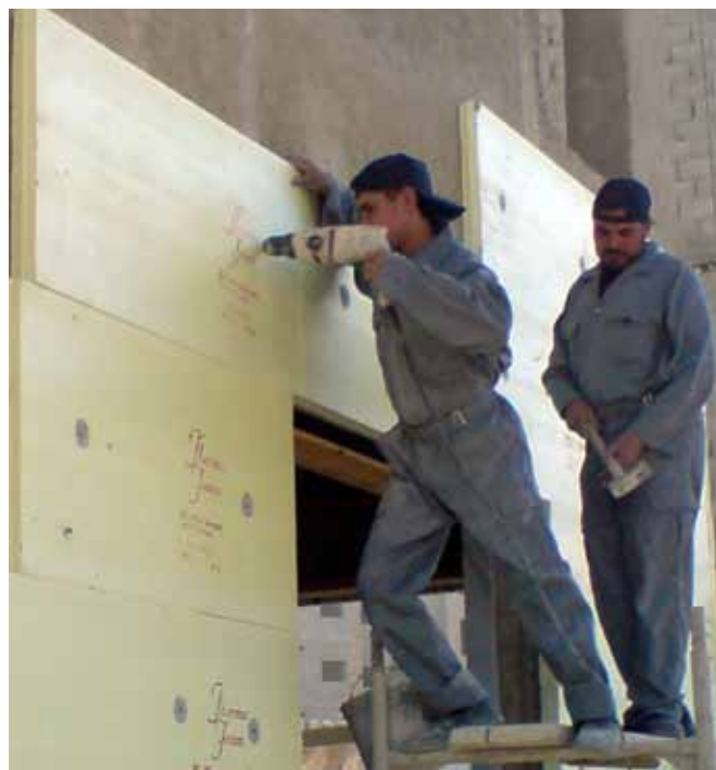
Applying thermal insulation on new buildings - Syria
