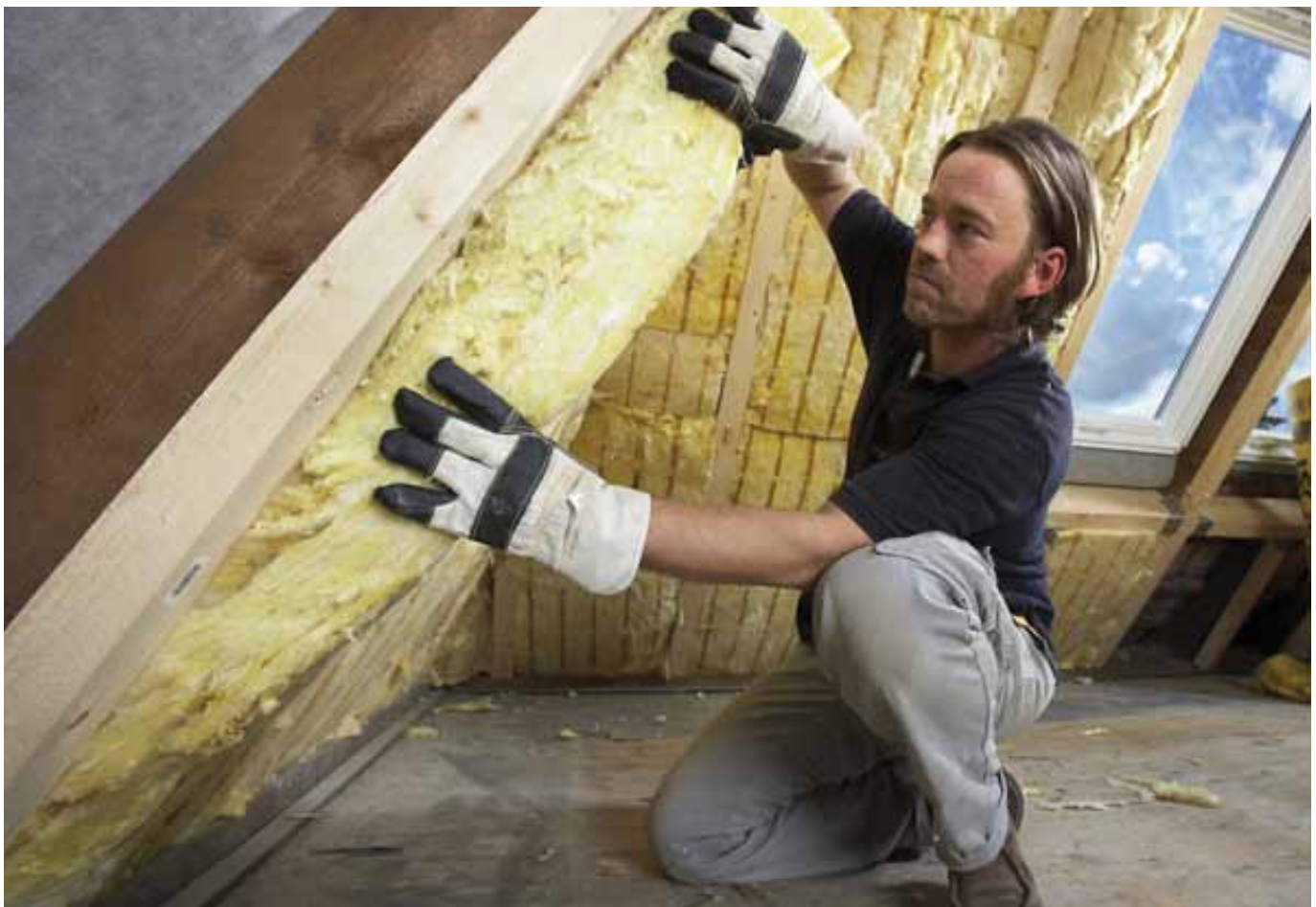
Applying insulation in the roof of an apartment
