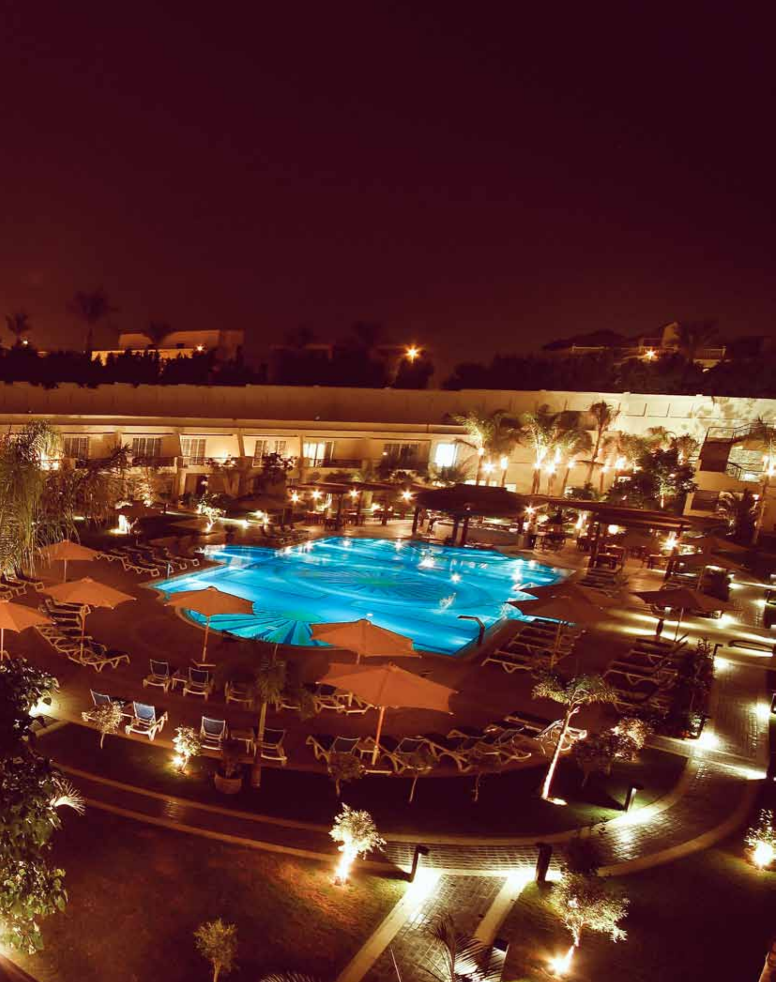
Energy Efficiency Lighting at Renaissance Hotel, New Cairo, Egypt
