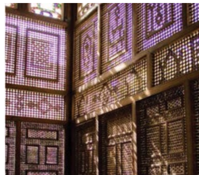
Mashrabeya traditionally are trapping cool wind keeping the heat outside such in this Bayt el Suhaymi house, Khan el Khalili in Cairo
