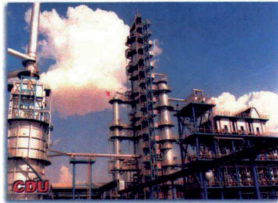
Crude distillation Unit (CDU)
