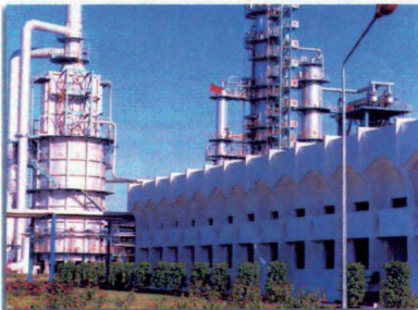
Distillation Columns Building (DCS) (Fractionator)
