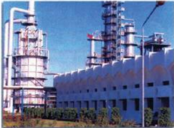
Distillation Columns Building (DCS) (Fractionator)
