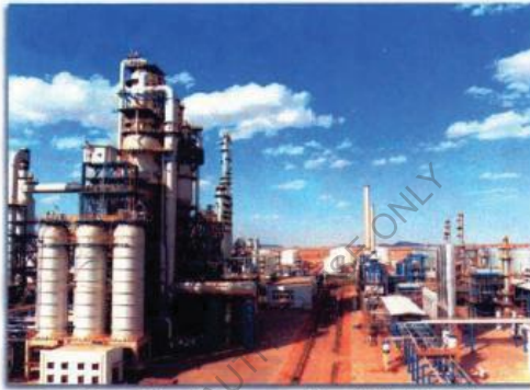
Residual oil catalytic cracking Unit (RFCC) . and Reforming Unit (REF)
