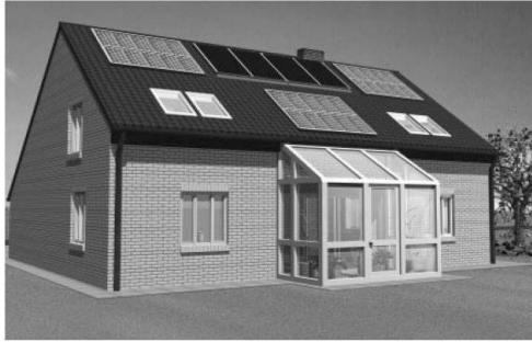
Figure 4.3. (Roaf, 2013). The first eco -house in the UK in 2013 showing the use of passive solutions with the solar energy system
