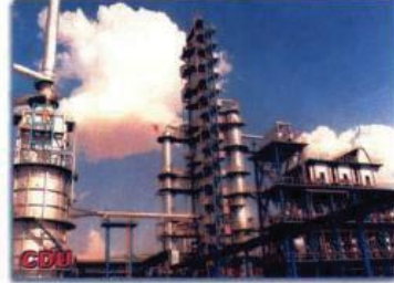
Crude distillation Unit (CDU)
