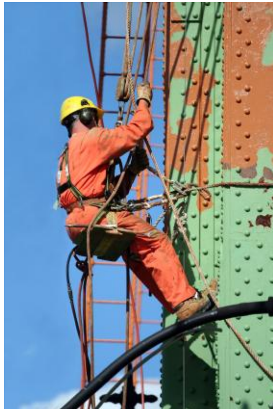
Figure 3.5 Correct use of lifelines and safety harness
