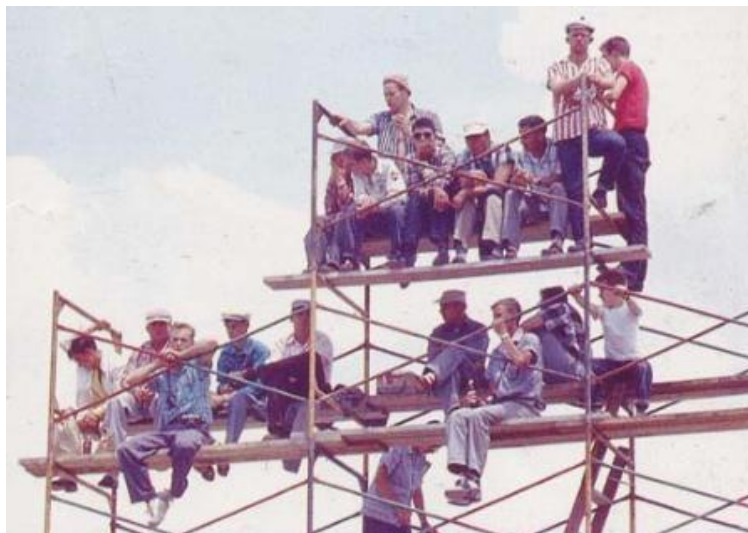
Figure 3.4: Incorrect Use of Scaffold
