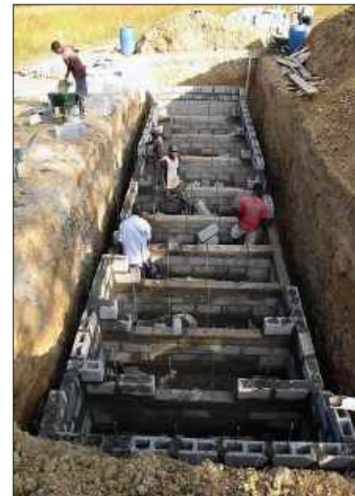
Fig(172): ABR being built in residential quarter in Zambia incorporation with German Toilet www.germantoilet.org/
