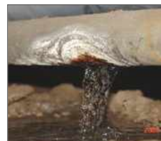
Fig(41) :Physical losses that cause (NRW).
