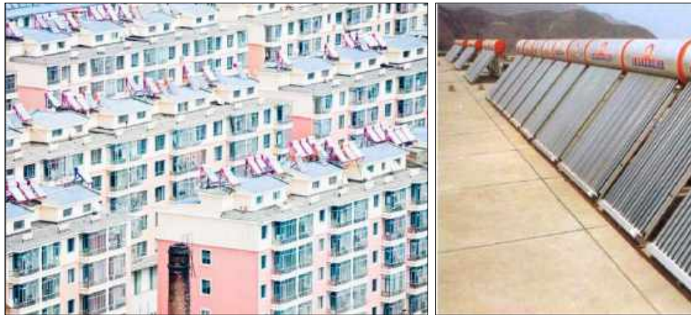
Fig(223): (left) Solar water heaters on newly built apartment blocks in Hunchun, China (right) Roof use for solar collectors - Source: (left) UN-Habitat/Alessandro Scotti (right) www.solarcities.com
