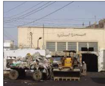
Fig(295): The main Municipality Garage of Tanta located in Ganabeya
