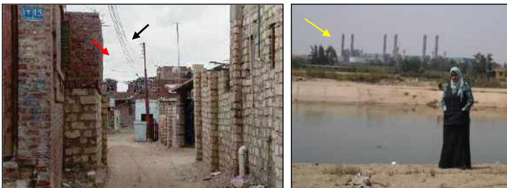
Fig(275): (left) Aerial electric cables serving Natrun houses (right) The researcher standing by Nubareya Power Plant supplying Natrun City, April,2015
