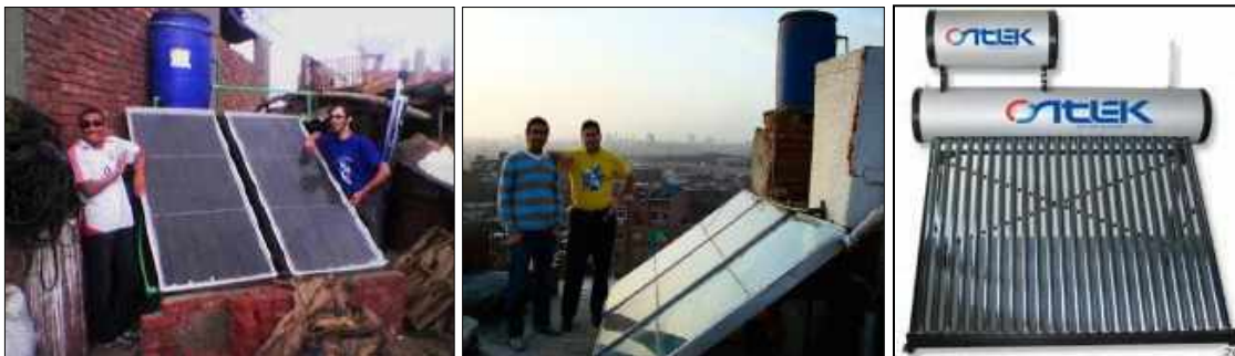
Fig(222): Locally made solar collectors above the roof of Zabaleen informal school (left) and in Historical Cairo (middle)- (right) An example for prefabricated solar collector. Source: (left) Photo courtesy to T.H.Culhane, www.solarcities.blogspot.com/ (middle) http://news.nationalgeographic.com/ (right) http://www.alibaba.com/ retrieved in 13/12/2015
