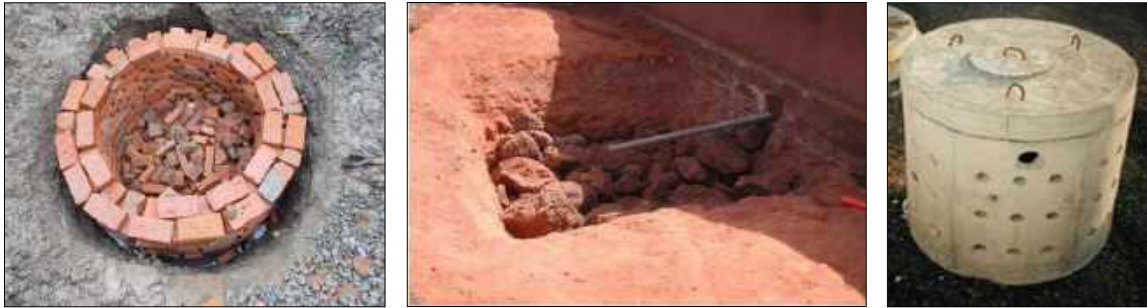
Fig(186): (a) Soak pit built in site (b): Open Soak pit (c) Prefabricated concrete pit (a) http://2.bp.blogspot.com (b) AHRENS (2005) (c) http://www.sswm.info
