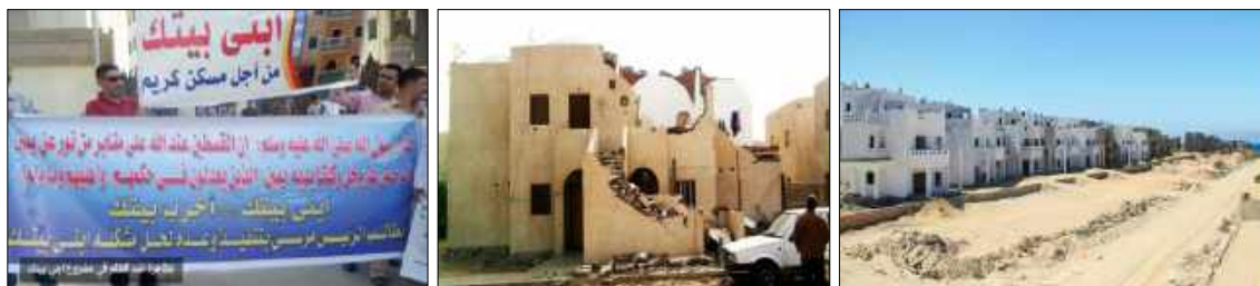
Fig(7) (left) Demonstrations against lack of utilities in Ebni-Beitak (middle) Dilapidated houses in Haram City (right) Vacant summer houses in the north cost.
