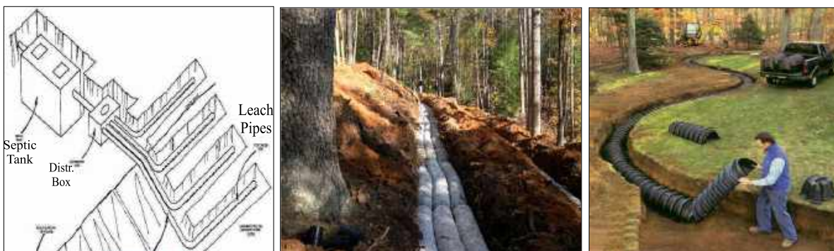
Fig(183): Leach field compatibility with different contours (b) gravel-free leaching system installed in North Carolina, USA (c) Prefabricated leaching system installed in Lancashire, UK.
