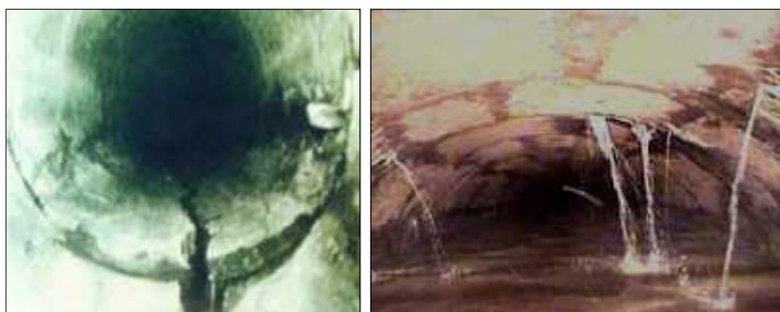
Fig (44): (left) Leaks from water and wastewater pipes into groundwater (right) Infiltration into water and wastewater pipes from the surrounding groundwater (right)
