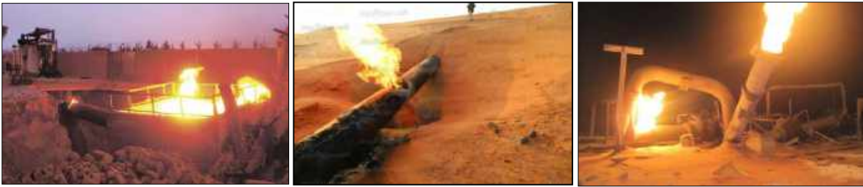
Fig (127): Recurrent Natural gas lines attacks in different locations in Egypt
