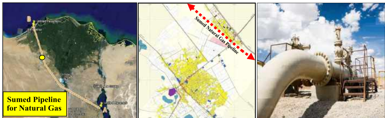
Fig(276): (left) Sumed Natural Gas pipeline path (middle) Sumed path across Natrun city (right) Gas pipes affecting the natural habitat of the area.
