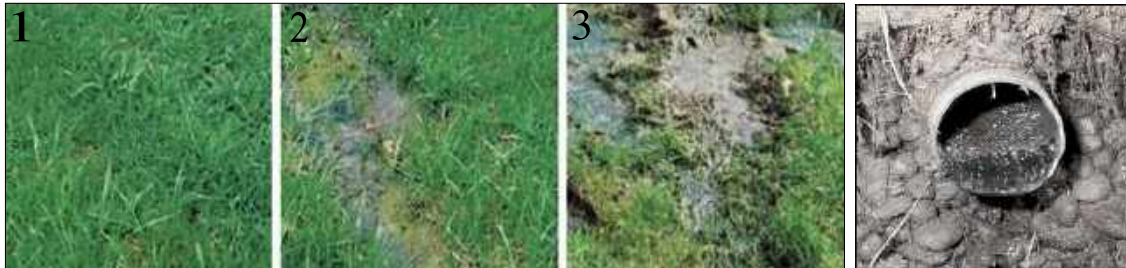
Fig(181): (a,b&c) Signs of failure of leach field system (d) Leaching pipe clogged with sludge due to insufficient primary treatment
