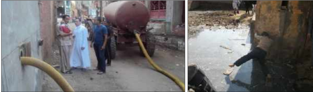
Fig(55): (left) Evacuation of rural trenches in Met Nama, Qaliubeya (right) Trench flooding in Afeih, Helwan
