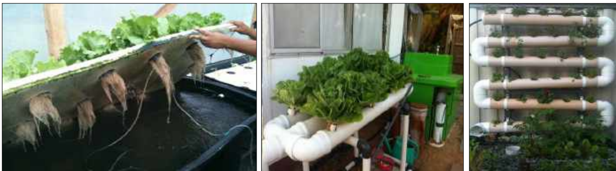
Fig(195): (a) Wetland cell serving a house in Thailand (b&c) Vertical & horizontal wetland systems installed through perforated pipes for residential wastewater treatment
