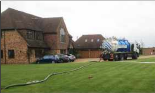
Fig(167):S.Tank pumping in London http://weatherheadgroup.co.uk/
