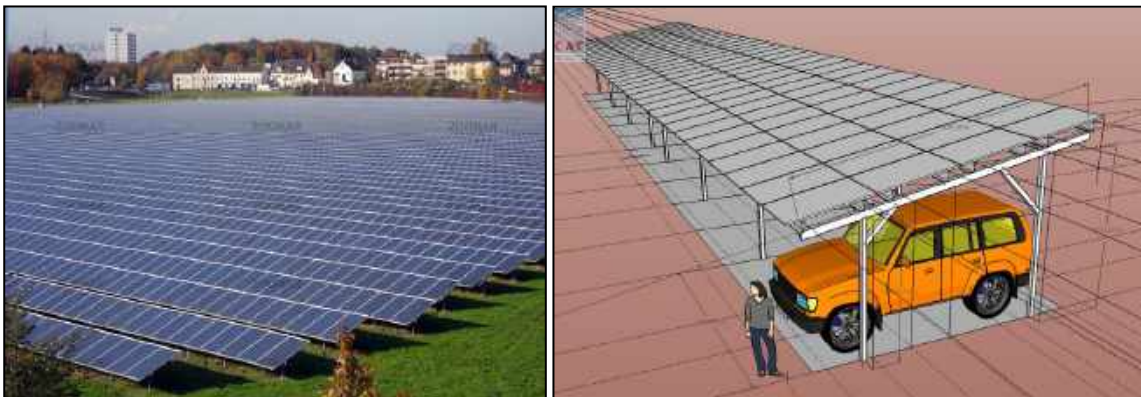
Fig(214): (left) Solar farm land use in Berlin, Germany 2010 (right) Zero land use of solar panels by using them as parking roof
