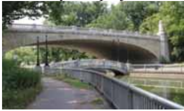
A bridge in Branch Brook Park, New Jersey accommodates multiple transportation needs- USA
