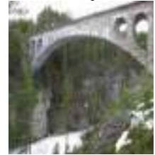
Wiesen Viaduct - Norway 3 - 54m
