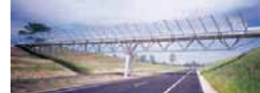
Structurally expressive form using modern materials is evident in this space-frame bridge- Australia
