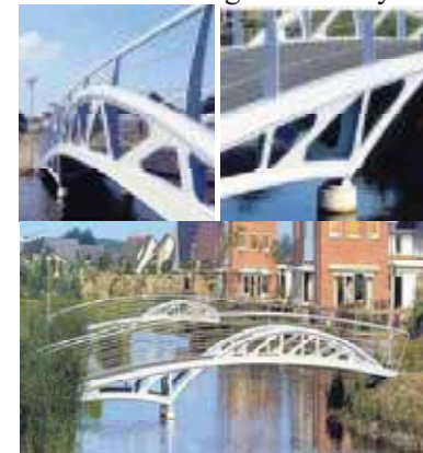
Emmeloord bridge, Netherland
