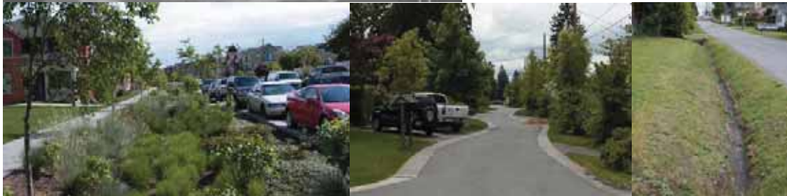
The High Point subdivision in the West Seattle neighborhood of Seattle, Washington: The grassy area (left) is actually turf placed over a large infiltration basin. A bios wale (center) is featured, and still in early growth. Alsoand the street (right) are paved with permeable concrete.
