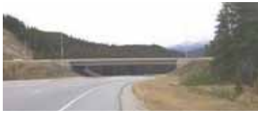
Bridge in Louise - USA
