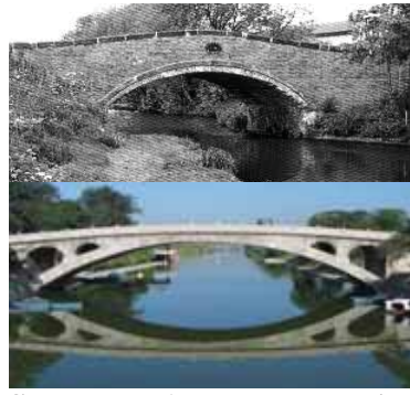
Segmental Arch: Segmental Arch Bridges- at China
