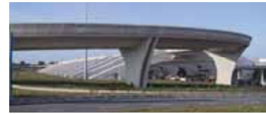
The horizontal and vertical geometry of the bridge have influenced the structural system selected for this bridge -Portugal
