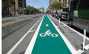
The green bike lane on Market Street approaching 10th Street. Photo: Bryan Goebel
