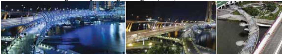
Figure 4-19: Example of pedestrian river front bridge (Helix bridge) 5
