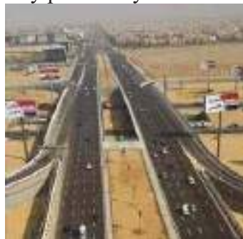
El-Mosher Tantawy bridge at Fifth settlement - Cairo - Was constructed to solve the traffic conjunction between ring road and ninety road 2
