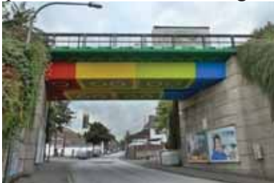
The Lego bridge in Wuppertal, Germany 3
