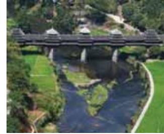
Chengyang Bridge, China
