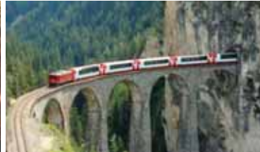
Landwasser viaduct, Switzerland
