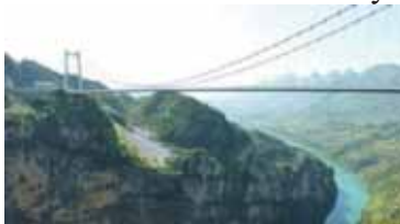
Beipanjiang River bridge
