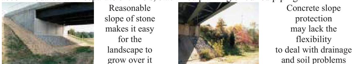
Figure 6-26: Slope Protection examples (in USA) 1
