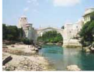
Bridge in Herzegovina
