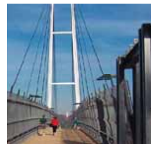
Dean Street pedestrian bridge in Albury. It forms one focal point of the Dean Street axis, the other being the memorial 5
