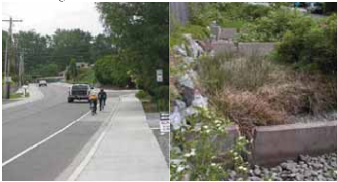
Washington. permeable pavement bikelanes -permeable sidewalk- A bioswale with flow control weirs.USA
