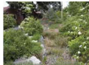
A well established vegetated swale/Bioswale that uses compost amended soil and no flow control devices or structures. Residential street to right. Seattle, USA / Greenroads
