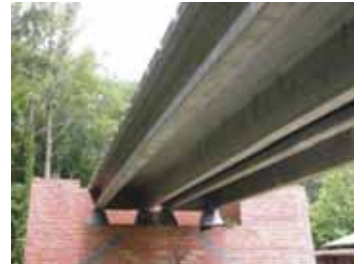
Test bridge using the fiber-reinforced cement composite, Virginia, USA 5
