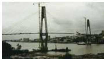
LRT Bridge across Fraser River in Vancouver is pleasing, long span cable-stayed bridge
