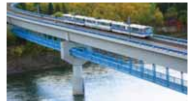
Railway bridge with a pedestrian path- Canada 5
