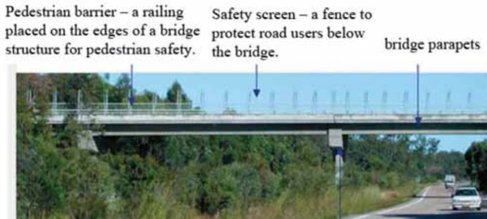
Figure 6-18: Bridge Non Structural Parts (by researcher)
