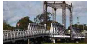
Modifications to Hinton Bridge over the Paterson River in Australia built in 1901
