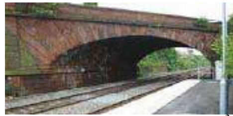
Skew Bridge : Rainhill Skew Bridge 3
