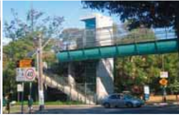
On the pedestrian bridge over The Boulevard in Strath field the placement of the girder to the side of the piers/ lift shafts allows for good district views out from the ends of the bridge.
