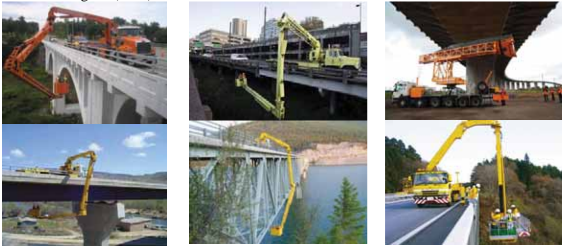
Figure 11-1: Examples on Bridge Maintenance Techniques 2
