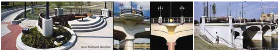
Figure 4-20: Pedestrian river front bridge (Bridge over Miami River Hamilton, Ohio) 6
