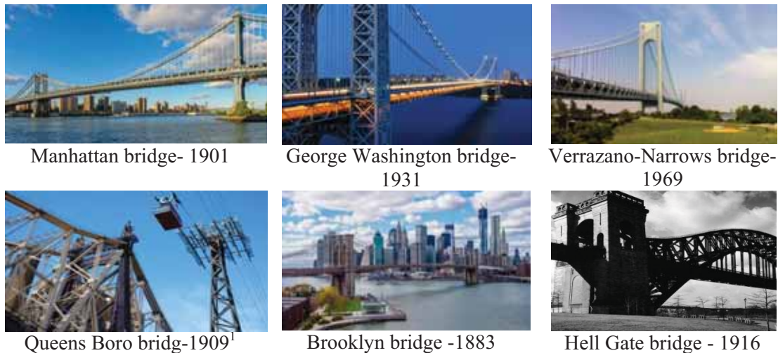
Figure 4-24: New York bridges as a city's landmark 2
