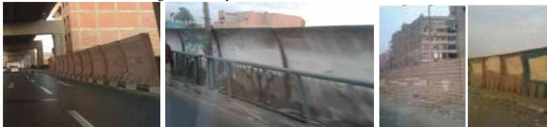
Ugly Noise walls at ring road - Saft ellaban corridor (by researcher)
