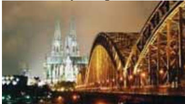
Hohenzollernbrücke Railway bridge, Germany
