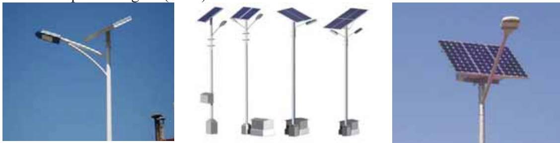
Figure A-12: Renewable energy luminaries at ring road /Cairo-Alexandria desert road
