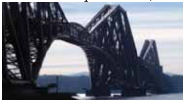
Forth railway bridge, Scotland
