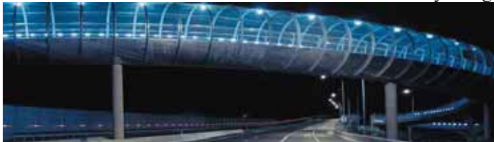
A bridge at Billinudgel uses the safety screen as a design feature, wrapping the whole girder and creating a distinctive tube effect.
