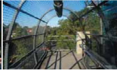
On the pedestrian bridge over The Boulevard in Strath field the placement of the girder to the side of the piers/ lift shafts allows for good district views out from the ends of the bridge.
