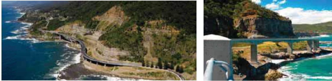
Sea Cliff Bridge - Australia (Spans proportions to height)
