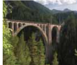
Wiesen Viaduct - Switzerland - 55m
