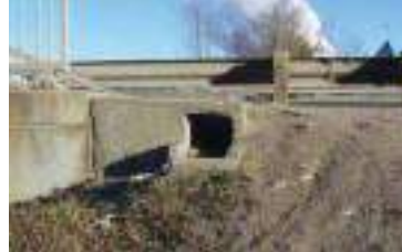
McLeod River Bridge At Whitecourt
