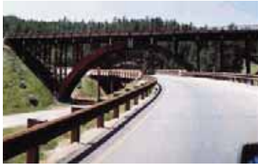
Natural beauty of site reflected in bridge type and materials, Black Hills National Forest, South Dakota
