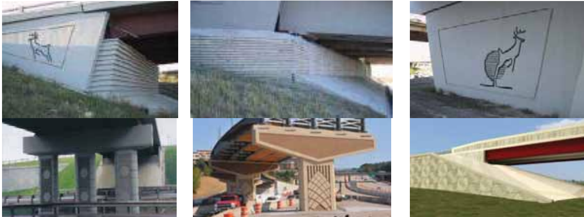
Figure 7-13: Concrete Patterns Examples (Different Bridges in USA) 2
