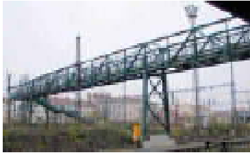
Truss girder footbridge Praha - Prague
