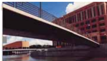
Steel box girder provides graceful, slender presentation, Rochester; Minnesota
