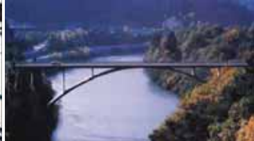
Having pedestrians on a bridge suggests the addition of overlooks. Upper Middle Road over 16 Mile Creek, Ontario.
