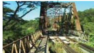
Abandoned Bridge in New Castle
