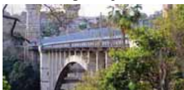
Distinguish new work from old Bridge, Australia
