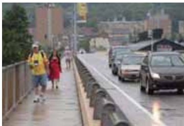
Fahy Bridge to get pedestrian lane next to unsafe sidewalks:
