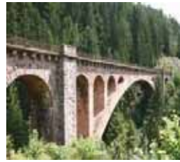
Gutach Bridge- Germany - 64m
