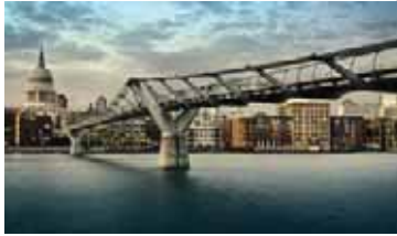
London Millennium Footbridge (2000) London,
