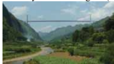
Baling River bridge
