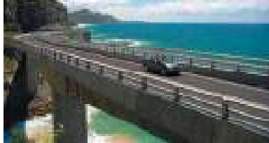
The sweeping form of the Sea Cliff Bridge, north of Wollongong, with two-rail parapet provides panoramic views
