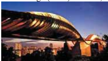
Henderson Wave bridge (2008) Singapore
