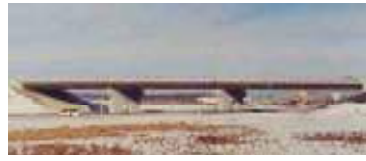
Mackenzie bridge - USA
