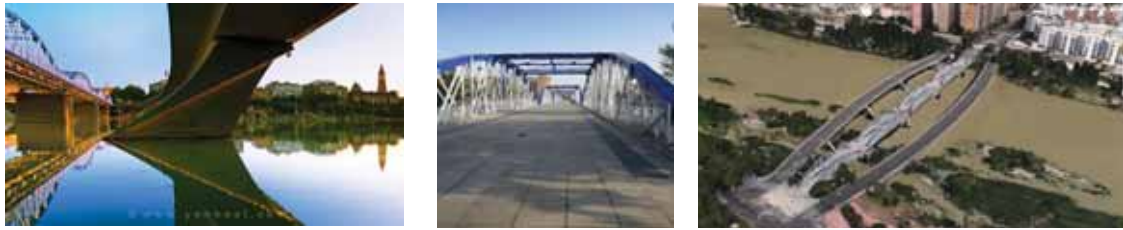
The Iron bridge in England was built in the late 19th century and remodeled in 1991. It has a central bridge for pedestrians and a vehicular bridge on both sides
