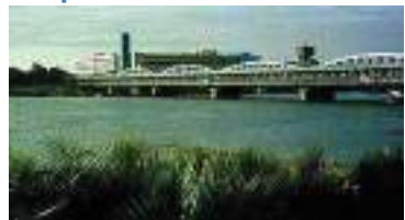
Imbaba multi usage bridge - Egypt 4
