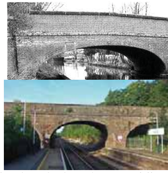
Semi-Elliptical Arch : Midhurst Road bridge, Lip hook 1
