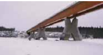
Peace River Bridge at Fort Vermillion - USA
