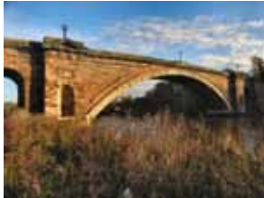
Grosvenor Bridge - UK 61m
