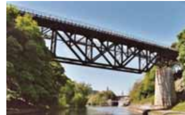
Deck truss railroad bridge over the Erie Canal
