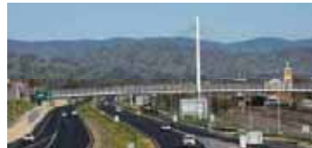
Using seven cables instead of three required structurally create an attractive Albury bridge
