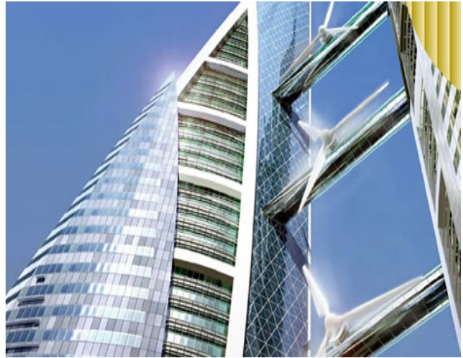
Fig (2-4) Bahrain World Trade Center Ref: Derek Markham. (updated 2020). Bladeless Wind Turbine Could Be 2X as Efficient as Conventional Designs.
