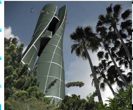
Fig (3-8) This structure was constructed to demonstrate how Nano Vent-Skin will be used for new design concepts.
