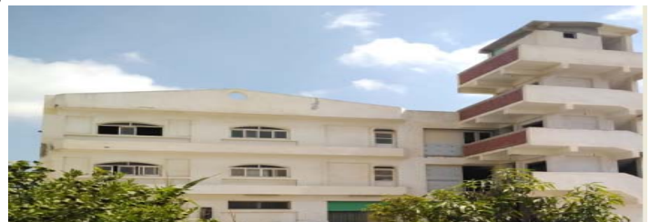
Fig (5-8) the Current building view
