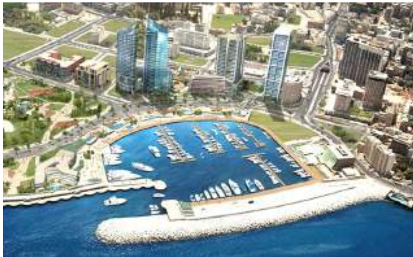
Fig (3-69) the Beirut Marina and the marina towers in the new waterfront.
