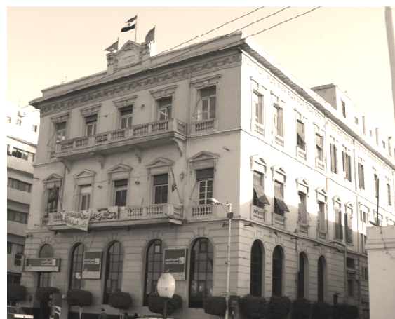
Fig (4-44) Mansoura municipality palace designed by an Italian architect A. Merrely
