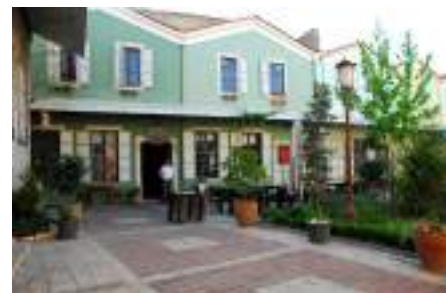
Fig(3-31) Abacioglu Inn after its transformation into a hotel.
