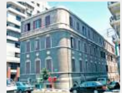
Fig (4-93) The prosecution's building characterizes by its Neo-Islamic style of its facades Source: (Researcher)
