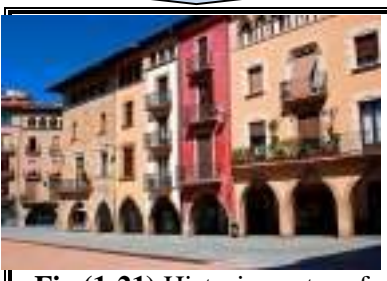
Fig (1-21) Historic center of c-Spain
