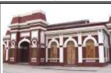
Fig (1-30) Old railway station currently being restored into a museum ,Granada- Nicaragua
