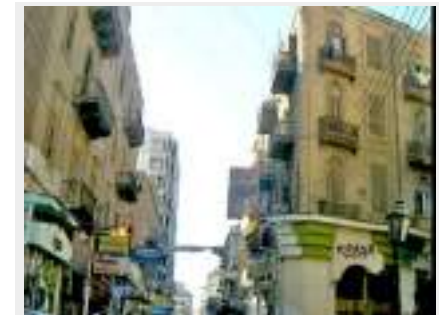
Fig (4-82) General view of the urban heritage site of eastern part of the sector(D). Source: (Researcher)
