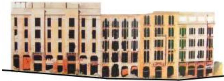
Fig (3-79) The west elevation of Allenby street before conservation process
