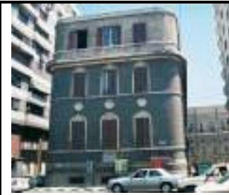
Fig(4-19) the prosecution's building (The Northern building of the khedive Ismail palace) Source: (Researcher)
