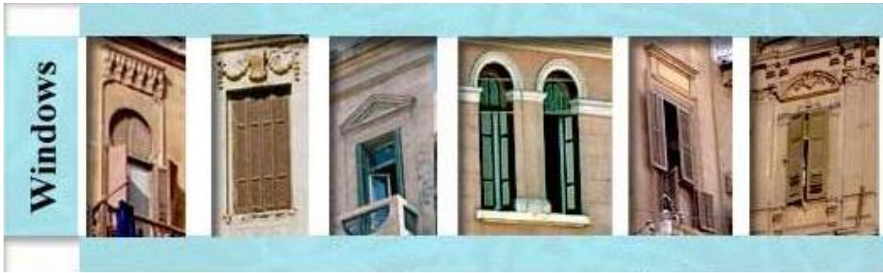
Fig (2-10). Some examples of the windows of El-Sekka el-Gedida street's heritage buildings at Mansoura city-Egypt, despite the different forms of them, the common feature is used the shutter windows for thermal comfort and privacy purposes.
