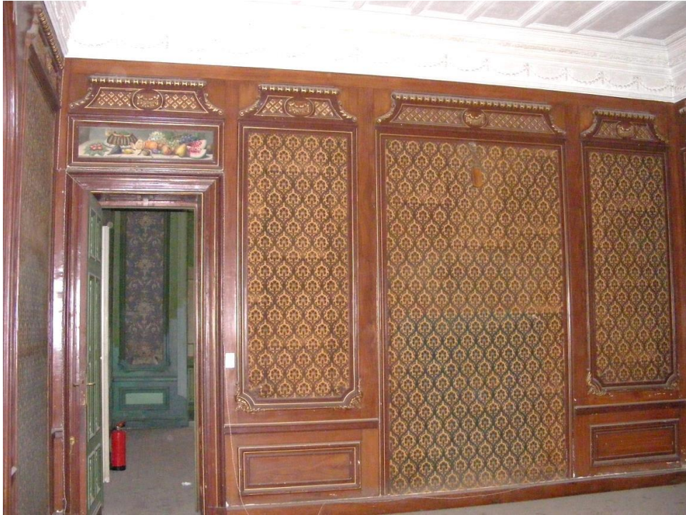
Fig (6-19). The dining room of El-Shenawy in palace the first floor
