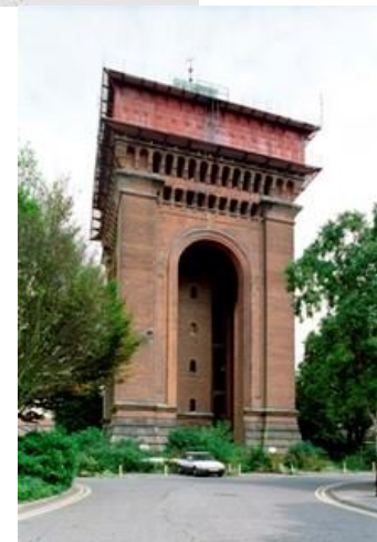
Fig (1-2). Municipal Water Tower -Jumbo, Colchester, Essex. Listed at Grade II Source: http://historicengland.org.uk/listing/selection-criteria/
