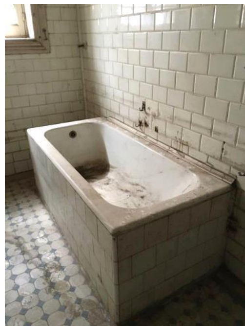
Fig (6-45). one of the bathroom of El-Shenawy Palace in ground floor
