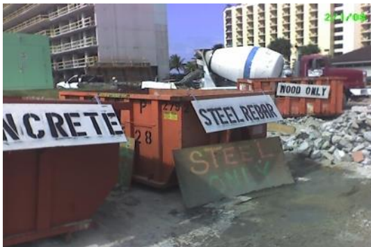
Fig (6-53), Three containers for site Materials waste
