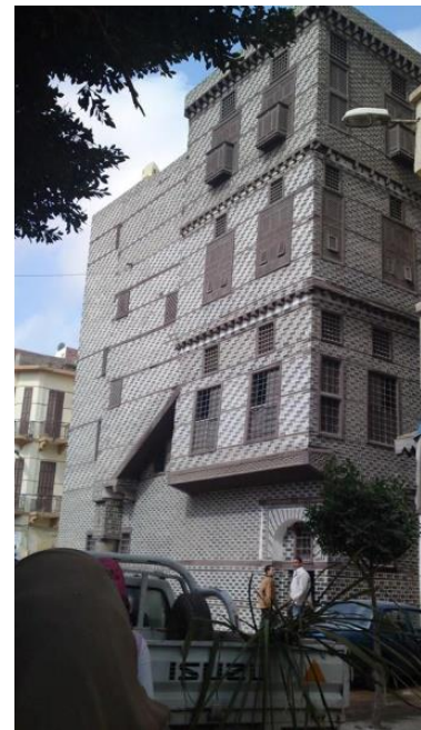
Fig (2-12) the skylight of the third floor's roof of Arab Kully's house in Rosetta-Egypt,
