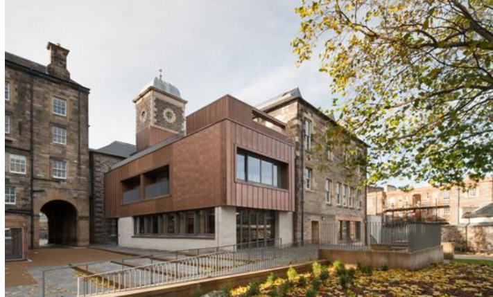
Fig (4-37). The side façade of ECCI building.
