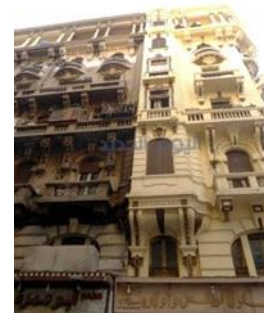
Fig (1-10). The painting works of a heritage building at Downtown-Cairo
