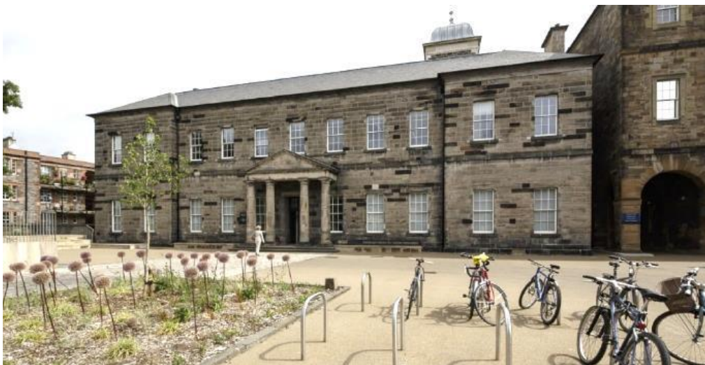
Fig (4-45). The bicycles racks in the front of ECCI building
