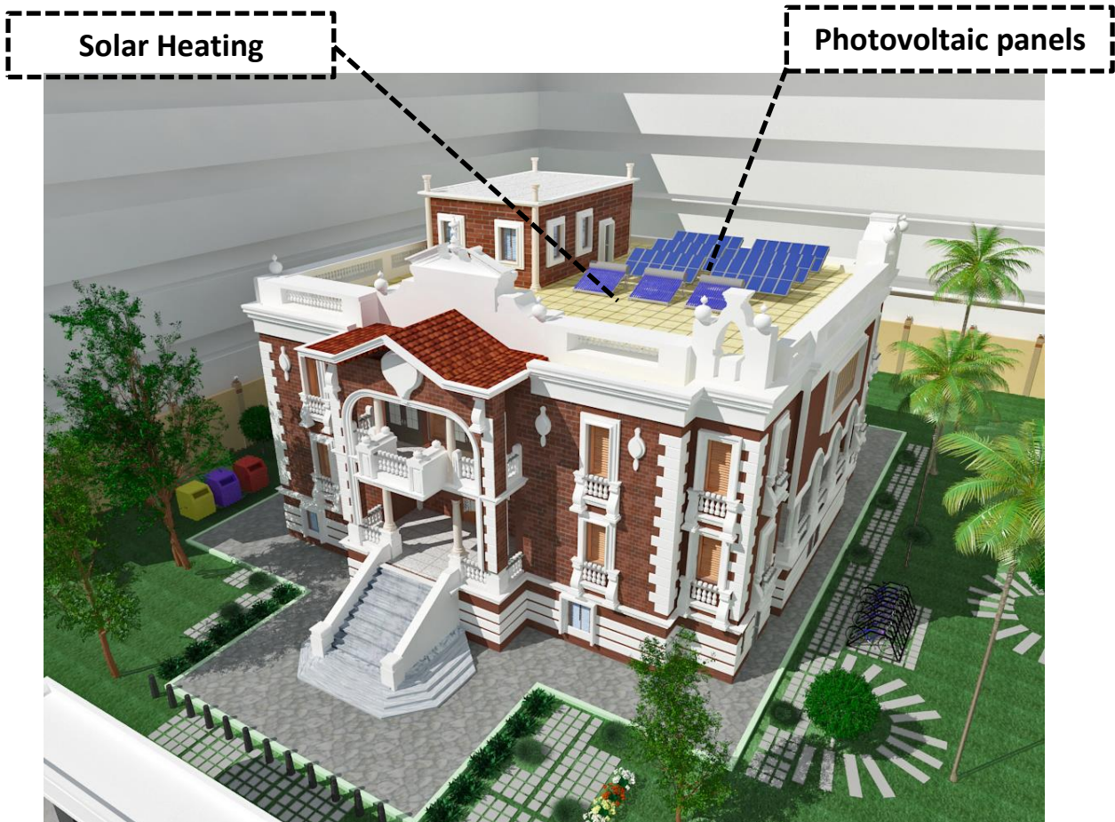
Fig (6-40). The location of the photovoltaic panels and solar heating system on the roof of the palace
