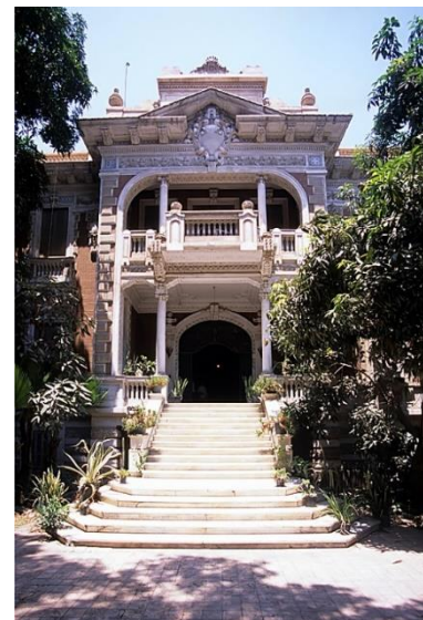
Fig (6-2). The main facade of El-Shenawy palace
