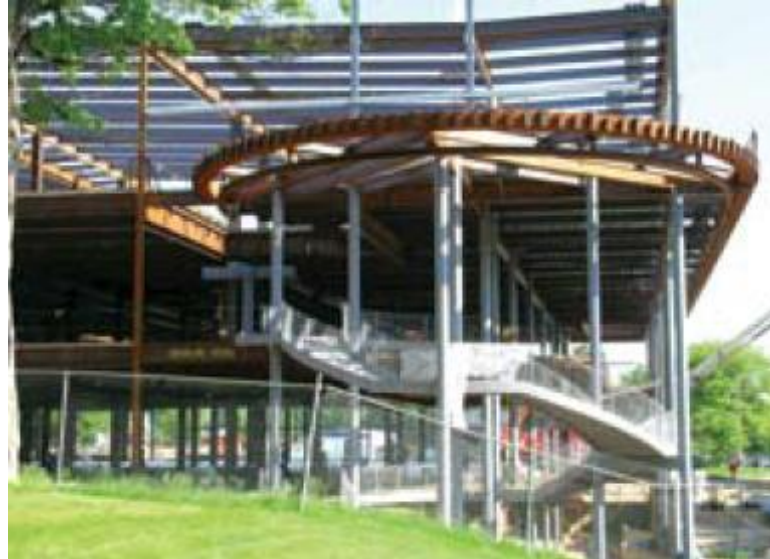
Figure 3.5: Health and Human Services Building during construction(Ruby, 2006)
