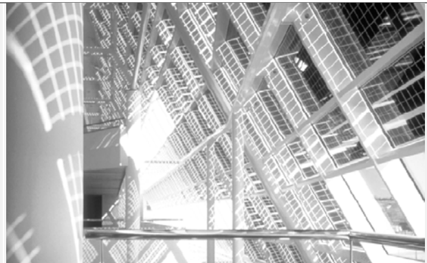
Fig. 2-52 Solar office in Doxford Sunderland (UK) with a transparent double glazing PV system integrated in the façade. Source: Maycock P, Schoen T, Strong S, Vigotti R, Reijenga T, et al, 'Building with PV.', (Ten Hagen& Stam,,1995)
