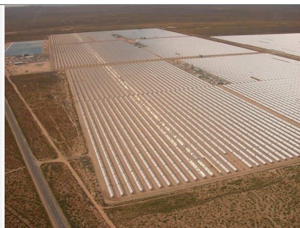
Fig. 2-2 Schematic View Of PLS- PV In The Desert illustrate to modular sets of 25MW unit Field. Source: http://en.wikipedia.org/wiki/Solar_power_plants_in_the_Mojave_Desert . Date. 1/2009.
