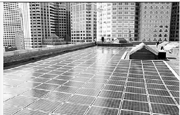
Fig. 2-50 Power guard flat-roof PV system including thermal insulation at the Coastguard building in Boston, Source: Eiffert P, Kiss G, " Building-Integrated PV Designs for Commercial and Institutional Structures " (NREL, Golden, Colorado 2000), 42-44.
