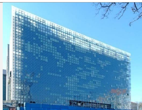
Fig. 2-54 The Largest Color LED Display Worldwide And The First Photovoltaic System Integrated Into A Glass Curtain Wall In China. The Building Performs As A Self-Sufficient Organic System Source: http://www.greenpix.org/project.php ,05/2008
