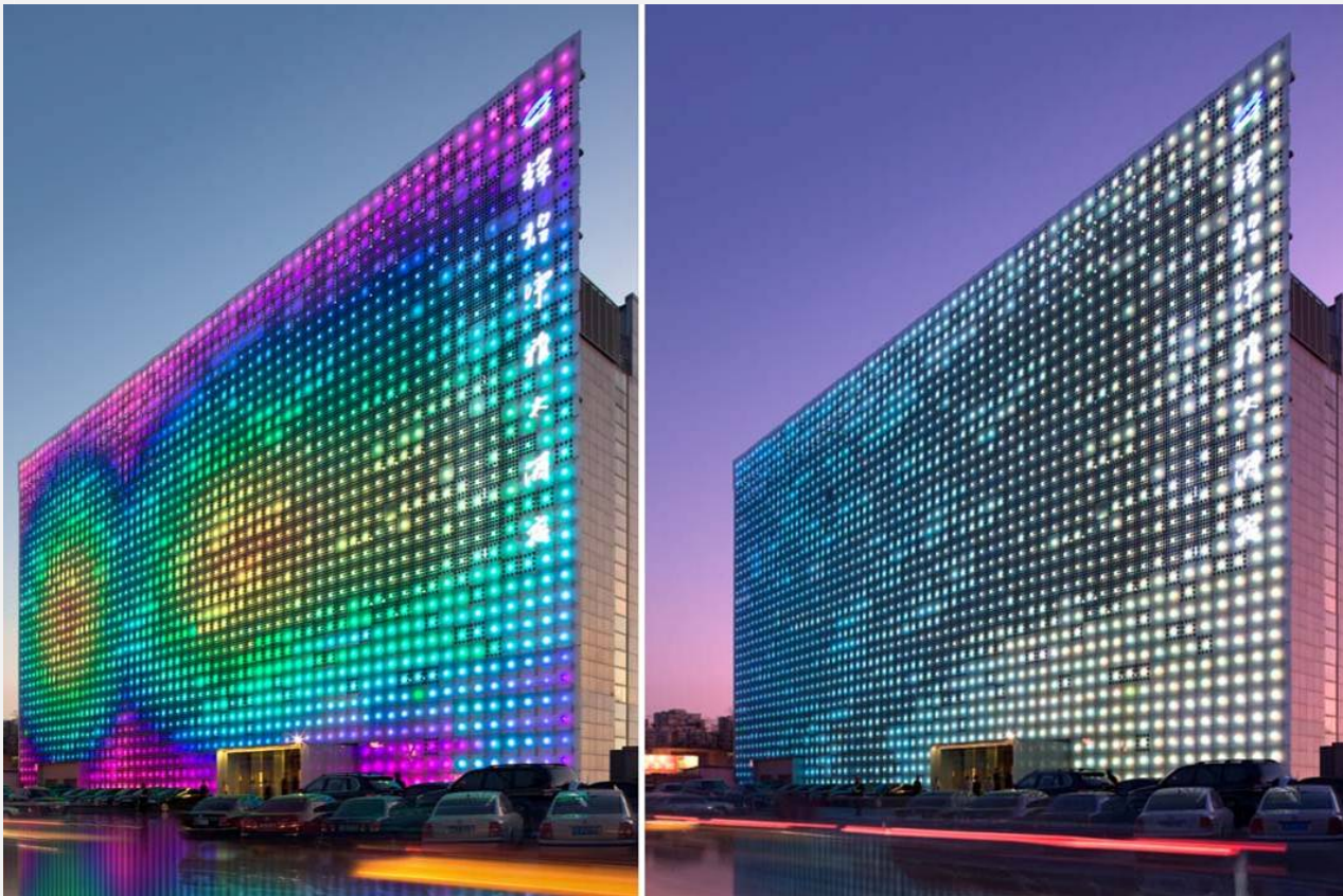
Fig. 2-56 The Largest Color LED Display And The First Integrated Photovoltaic System Into Curtain Wall, China, Source: Giostra, Simone, Arup, "Green Pix- Zero Energy Media Wall" http://www.greenpix.org . 05/2008.
