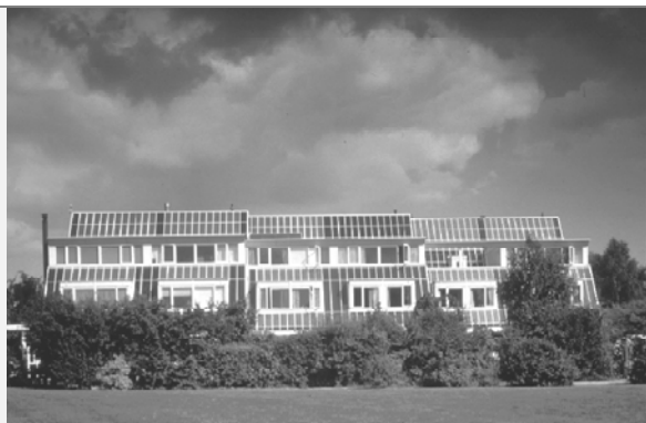
Fig. 2-49 Impermeable layer Roof integration, renovation project with the Shell Solar / BOAL profiles in Leiden (NL), providing a 2.1 kWp system per house. Source: Maycock P, Schoen T, Strong S, Vigotti R, Reijenga T, et al, ' Building with PV. ', (Ten Hagen& Stam, Den Haag, 1995) 78 – 81
