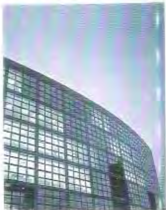
Figure 7.26 D.G Bank, Hamover, Germany by Bablo-Kolmke-Stosberg. A small panel size repeatedly used in the elevation, (Buton and Pys, 1993).
