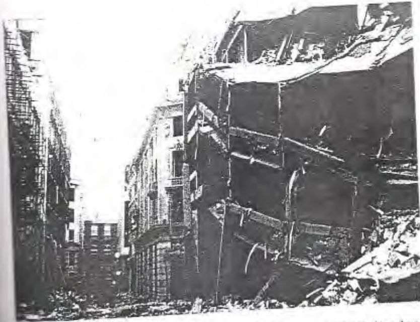
Figure 2.2 This view was taken of the area adjacent to the blast ( Times , 25.4.1993) looking along Bishopsgate. The severe structural damage in the near field is shown. Cladding strengthening would clearly bring no benefit close to the blast site.
