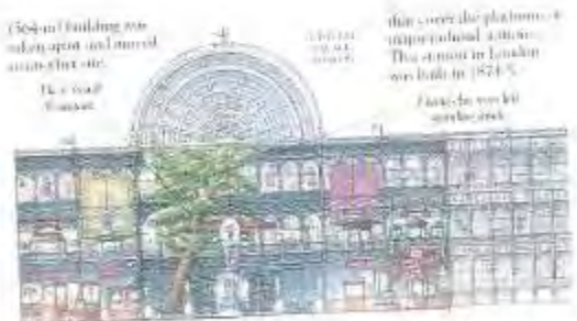
Figure 7.20 The Crystal Palace, London. The building built for the Great Exhibition of 1851, Paxton's Crystal Palace constructed with prefabricated cast iron parts and sheets of glass. It was built as an early form of temporary structure in order to be rebuilt for several times at different places
