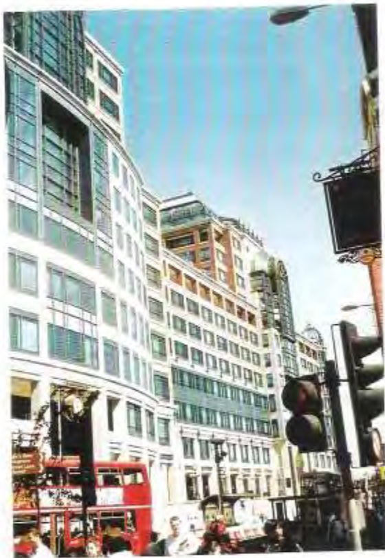
Figure 7.28 A typical building, Aldgate, London. The buildings have grouped areas of curtain walls together with solid material. This treatment increases the elevation's natural resistance.
