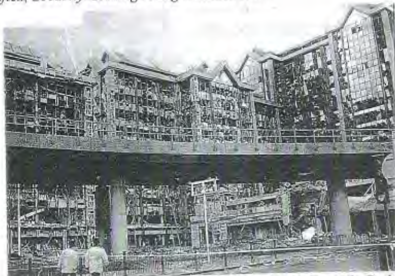
Figure 8.2 The use of laminated glass kept the glass in place when broken at the Docklands, ( Times, 1995 ).
