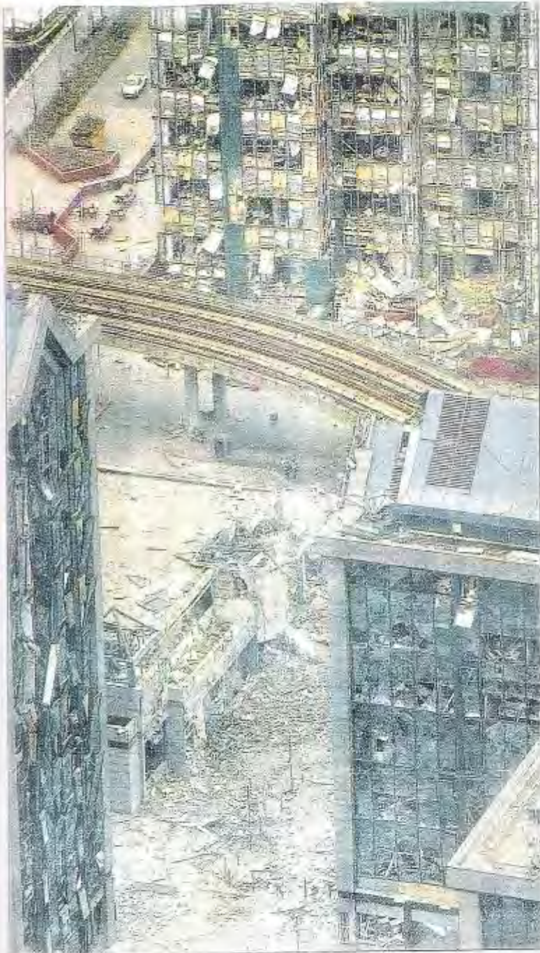
Figure 2.6 Most of the cladding materials within the bomb site need to be changed, ( New Civil Engineer , 15.2.1996).
