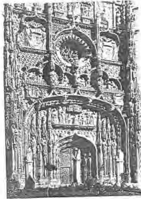
Figure 5.37 S. Pablo, Valladolid: principal doorway, J. Musgrove, 1989.
