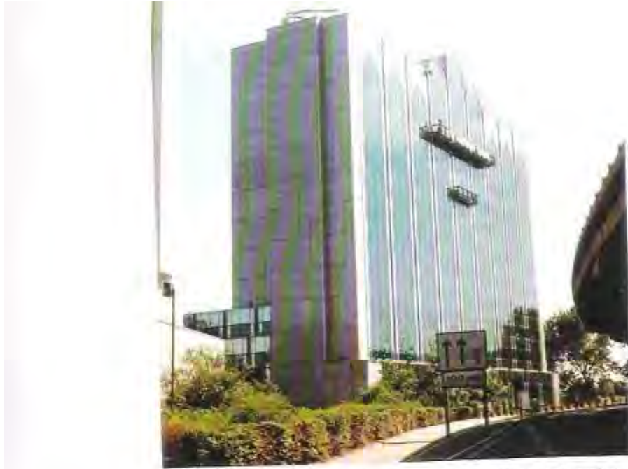
Figure 7.8 A typical example of curtain walling in London.
