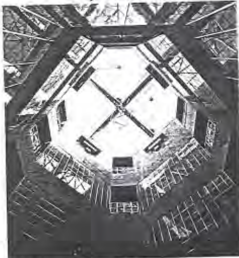
Figure 4.13.c Kisho Kurokawa, Saitama Museum of Art 1981-82, interior (Jencks, 1993). Using indoor open space it is advised to minimise the openings as shown.
