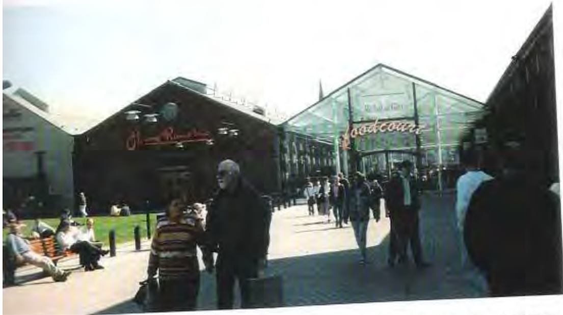
Figure 7.6 The entrance hall, Outlet Village, Swindon. The glass curtain wall used in the construction of a new building to integrate with old existing structures.
