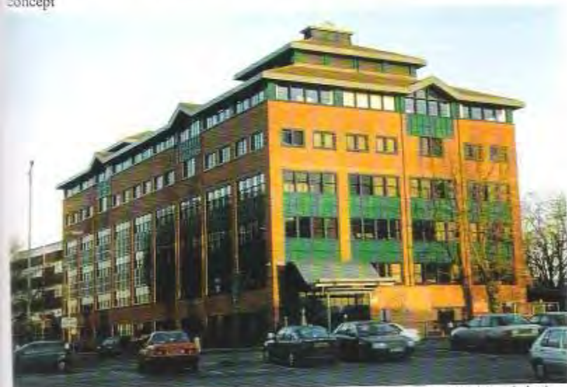
Figure 7.30 A typical office building, Swindon. In the elevation glass used with brick and plastic, reducing the area of glass increases the elevation resistance.
