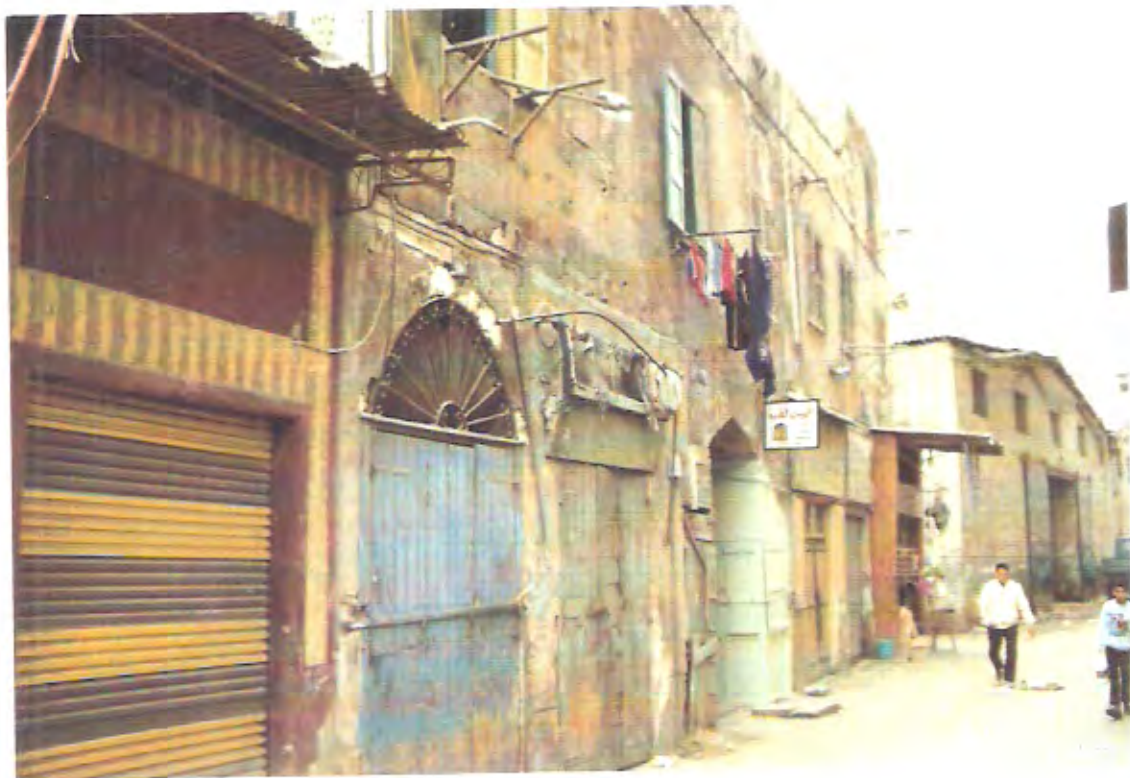
The building as seen from the street
