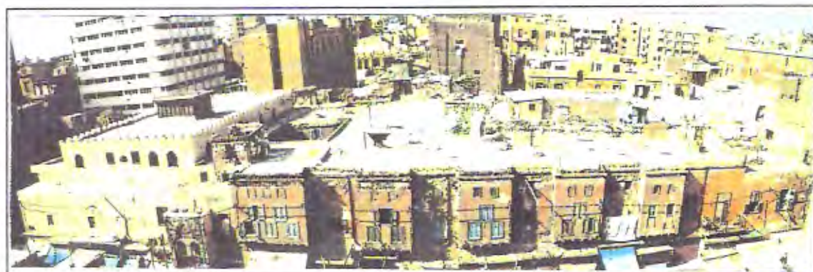
Fig.8-2, The building as seen from a higher blocks of flats; the southern facade: to the left, the mosque and its entrance; to the right, the wekalah : shops on the ground floor and five cells on the first floor.
