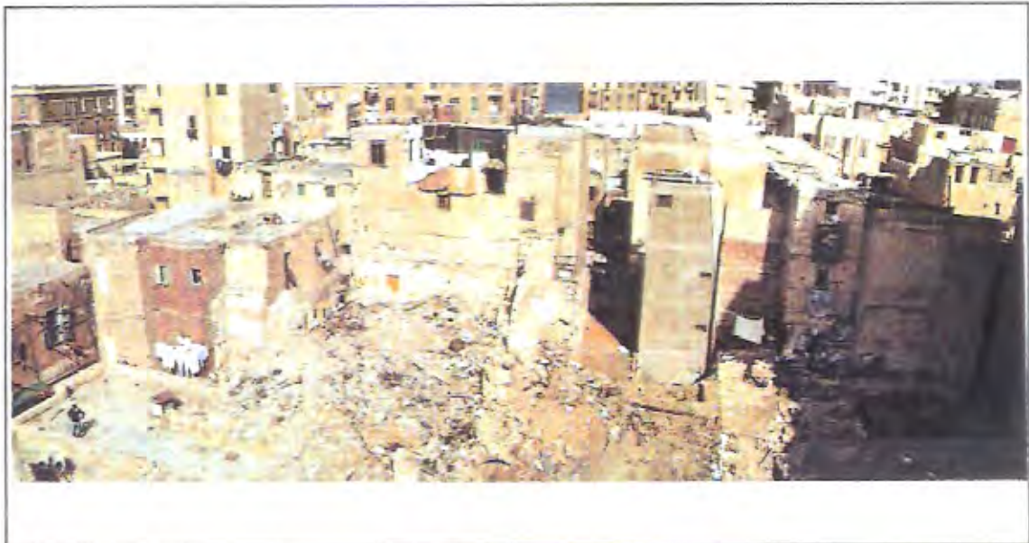
Fig.8-24, Waqf Gemaiee, the present condition: a real waste of resources
