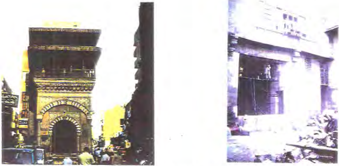
Fig.3-8, Involvement of foreign institutes in restoration; right: Sabil Abdurrahamn Kathkhuda restored by the German; left: Beyt Assit Wassila being restored by the French.
