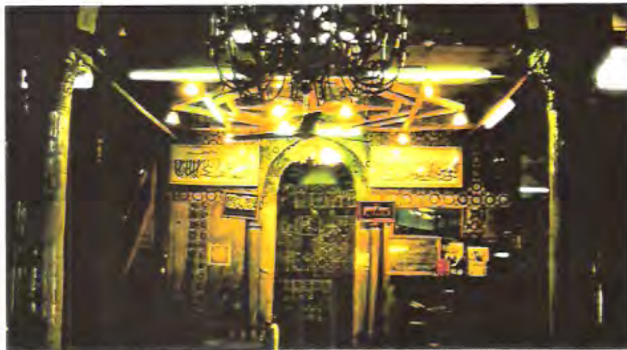
Fig.5-34, the interior of Terbana mosque; unsympathetic fittings to the original fabric.
