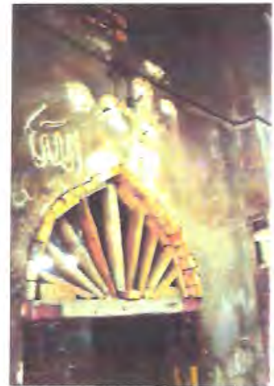
Fig.3-7 Right, Buildings were seriously damaged; not all resulted from the Earthquake. Left, Emergency scaffolding has been erected to support threatened structures; the efficiency of this questionable.
