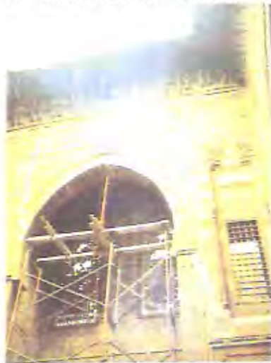
Fig.3-7 Right, Buildings were seriously damaged; not all resulted from the Earthquake. Left, Emergency scaffolding has been erected to support threatened structures; the efficiency of this questionable.
