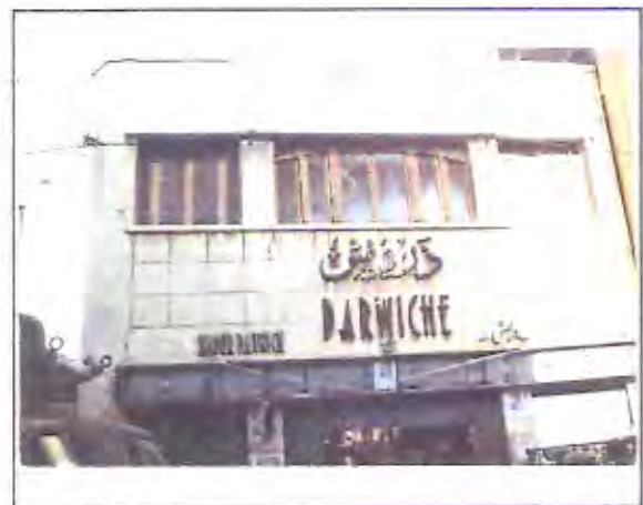
Fig.8-18, the street facade; a unique example of very "early-modern" architecture in Alexandria
