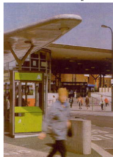
Figure (2-37), new facilities should provide passengers with facilities and response to the microclimate.
