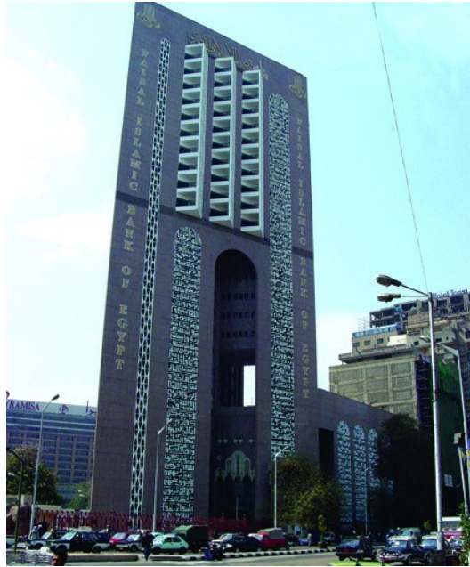
Figure 2-10 picture showing the north façade of Feisal Islamic bank and it's lattice screen
