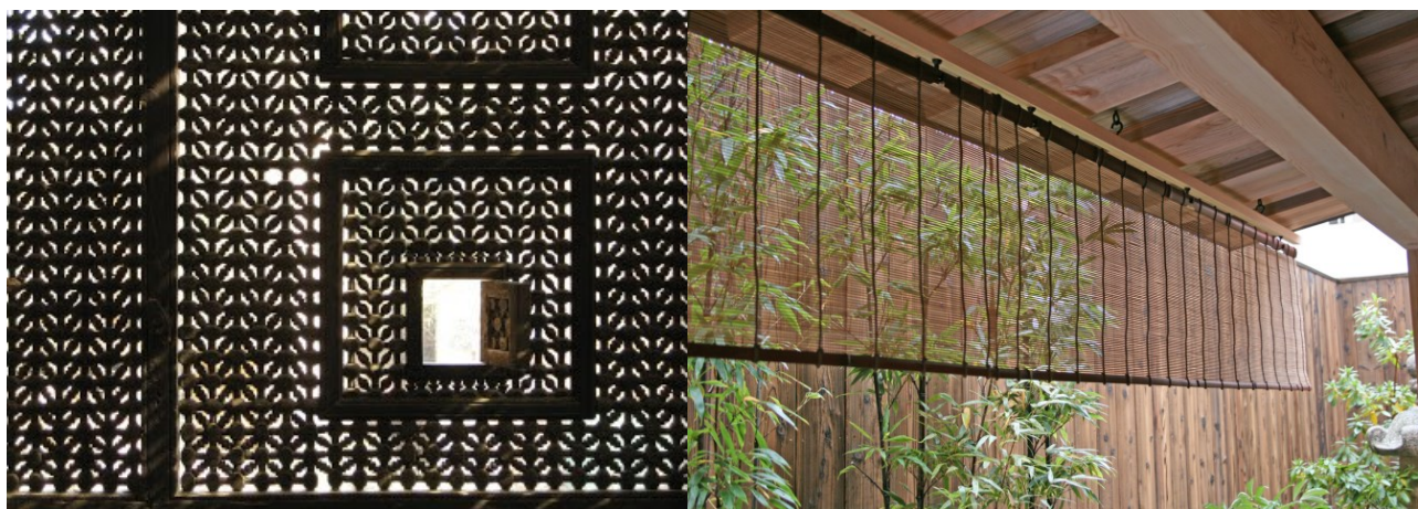
Figure 2-9 Different types of traditional lattice screens in Egypt mashrabiya (left) and Japan’s sudare(right) (source (Satoh Blog , 2011))
