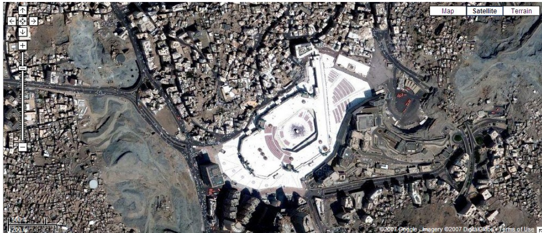
Figure (3-15/c): Compact grid with route pattern around Al-Masjid Al-haram, Makkah, Saudi Arabia
