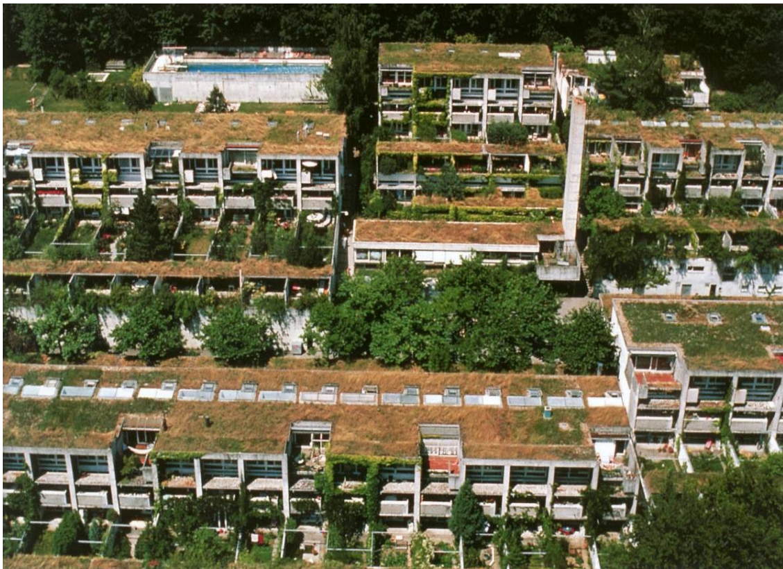
Figure (2-7): A combined passive techniques; array of green roof with a remarkable green back yard in completion with adjusted fabric form and orientation, adopted from (Herzog 1996 ).
