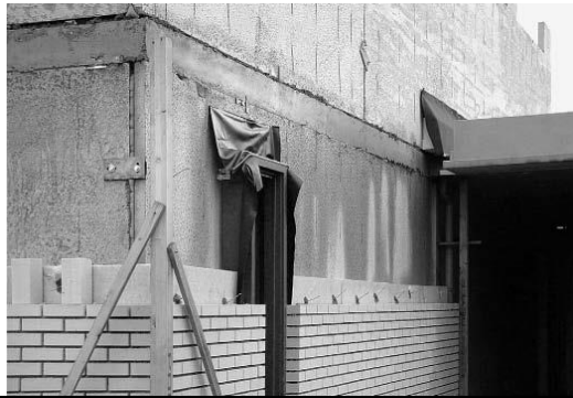
Fig.2-10:Masonry cladding taken from a housing development in Middelburg, the Netherlands
