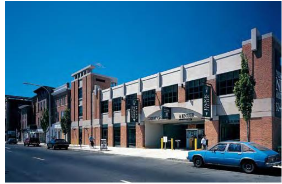
Fig. 1-17: The Ninth Square, New Haven, Conn. Source: http://www.sustainableprecast.ca/downloads/Precast_Achieves_Sustainability_Goals.pdf
