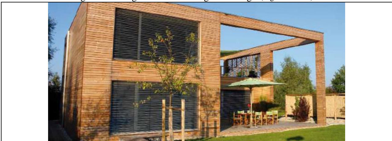
Fig. 4-26: Building façade with wood cladding
