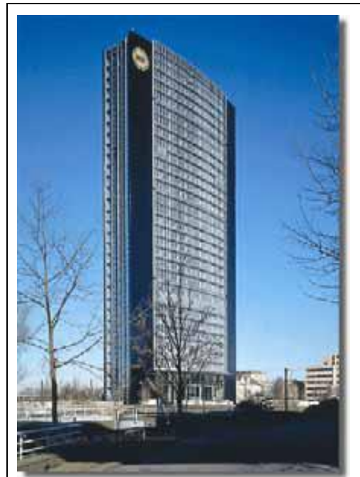
Fig. 3-7: View of ARAG 2000 Tower
