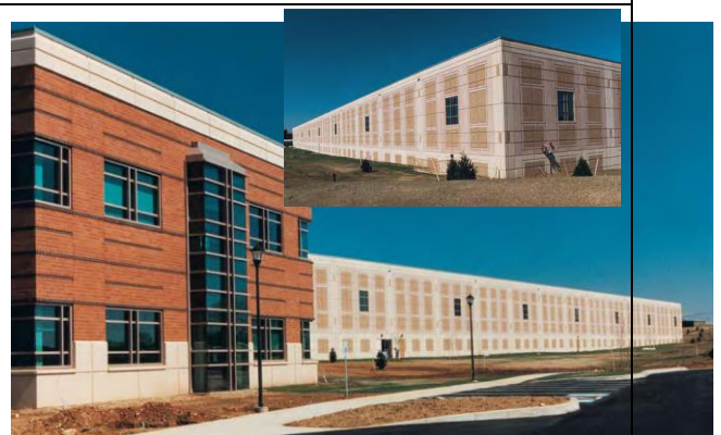
Fig. 1-21: Phillips Communications, Lancaster, Pa. Source: http://www.sustainableprecast.ca/downloads/Precast_Achieves_Sustainability_Goals.pdf
