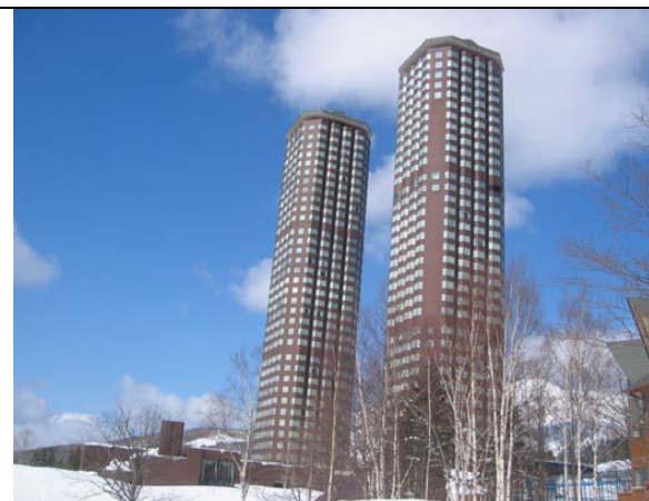
Fig. 3-54: Tomamu towers before re-skin
