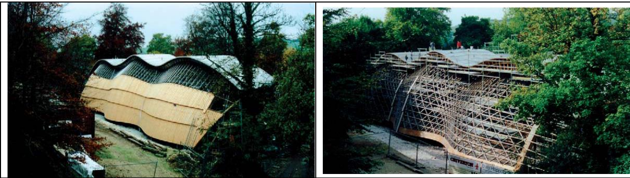
Fig. 1-8: Gridshell construction – Weald and Downland Open-Air Museum. Architects: Edward Cullinan Architects
