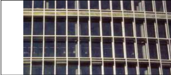
Fig. 3-8: View of the façade
