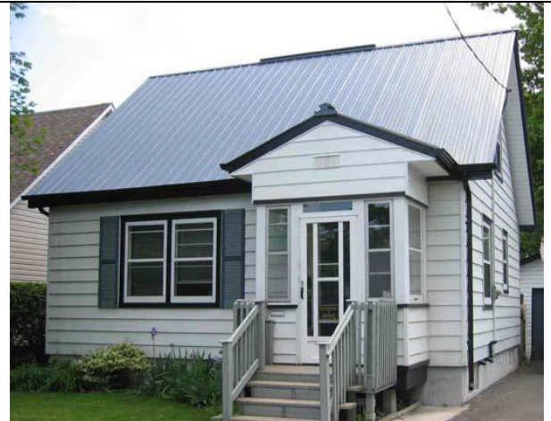
Fig. 3-46: Now house before re-skin
