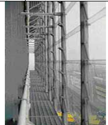
Fig. 3-15: Cavity of Debis headquarters
