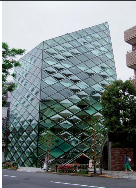
Fig. 1-27: Curved rhomboidal glass panes – Prada Store, Tokyo. Architects: Herzog and de Meuron.
