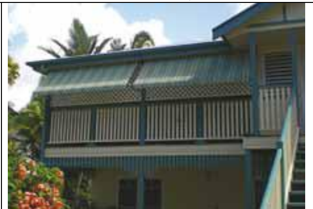
Fig. 4-2: Adjustable shading
