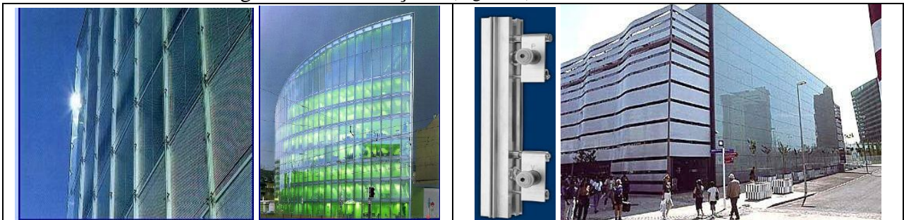
Fig. 4-7: Transfer the façade into double skin Source: Butterworth-Heinemann, Intelligent skins, Michael Wigginton and Jude Harris 2002, p.125
