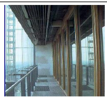
Fig. 4-16: Shaft-box façade
