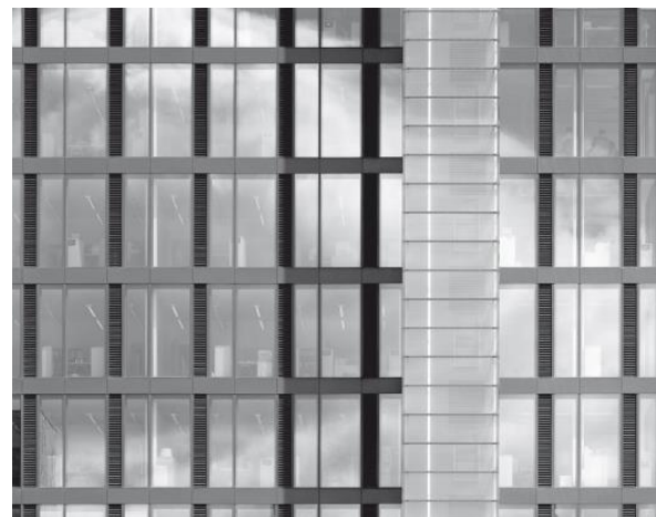
Fig.2-26:Debitel Headquarters, Stuttgart, RKW Architektur + Stdtbau, 2002
