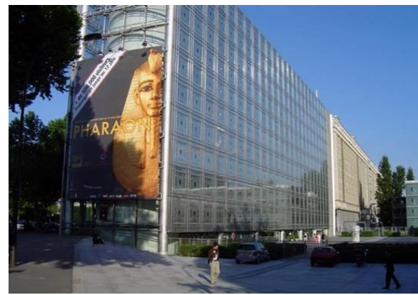
Fig. 3-21: The South-west facing walls
