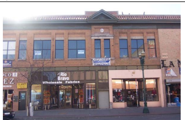
Fig. 4-4: Reflective glass Source: Kathy Dodson, Commercial Façade Improvement Grant Program Guidelines, 2009,
