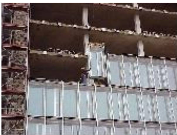
Fig. 1-47: Assembly of box double-skin façade units
