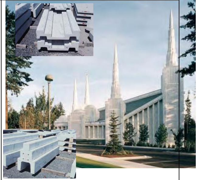
Fig. 1-19: Church of Jesus Christ of Latter-day Saints, Lake Oswego, Ore. Source: http://www.sustainableprecast.ca/downloads/Precast_Achieves_Sustainability_Goals.pdf
