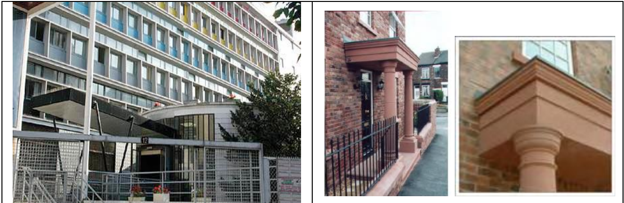
Fig. 4-31: Pre-cast concrete units for solid parts of façade
