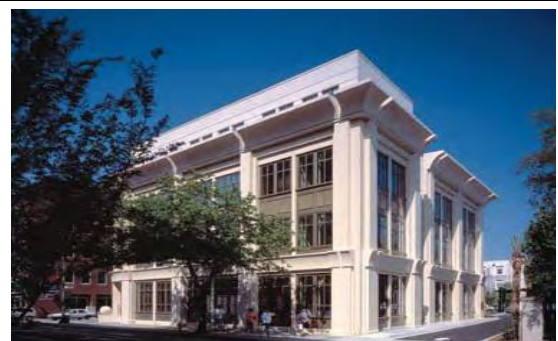
Fig. 1-15: South Trust Bank of Charleston, S.C.
