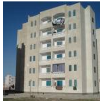
Figure 1-16: Al-Talet prototype ( National housing project )
