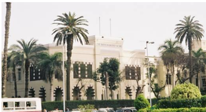
Figure 6-1 The American University of Cairo (Tahrir Campus) (Source, (aucegypt.edu, n.d.)
