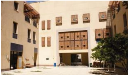
Figure 6-25 Louis Greiss courtyard in Abdul Latif Jameel Hall- zone B- AUC campus (Source, aucegypt.edu, n.d.)
