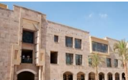
Figure 6-27 The open glazing windows in the north-east elevation of the school of business- zone B- AUC campus (Source, aucegypt.edu, n.d.)
