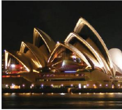
Figure 2-2 The “wings” of the Sydney Opera House (Kellert and Calabrese, 2015)
