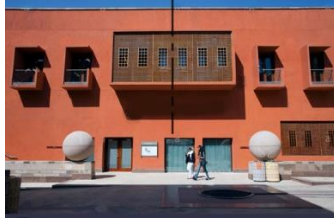
Figure 6-66 Symmetrically designed façade- student campus- zone B- AUC campus (Source, Edit by Author)
