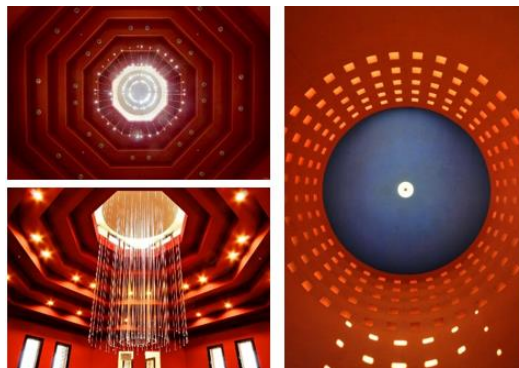
Figure 6-33 Shakhshikha and clerestories in zone C- AUC campus (Source, arch.egy, 2016)
