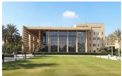
Figure 6-30 The open glazing windows in the north-east elevation of the main library- zone B- AUC campus (Source, aucegypt.edu, n.d.)
