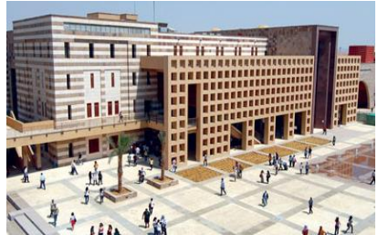
Figure 6-29 The shading devices in the south-west elevation of the main library- zone B- AUC campus (Source, aucegypt.edu, n.d.)
