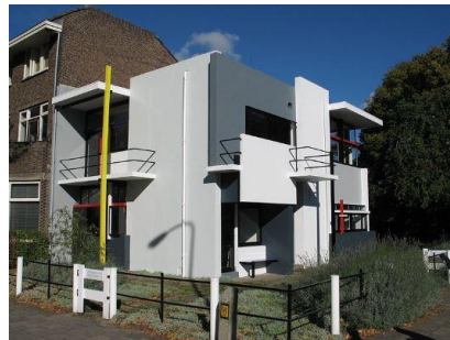
Plate 13 G. Rietveld and T. Schroder: Schroder House at Utrecht. 1924- Concrete, brick, and plaster, wood, steel girders –Utrecht, The Netherlands
