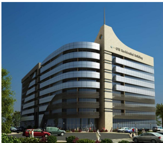
Fig (13): Above, Perspective for QIB proposed by ECG, & Designed by Dr.Wael Abo Neama, Below, on the other side Thermal loads study
