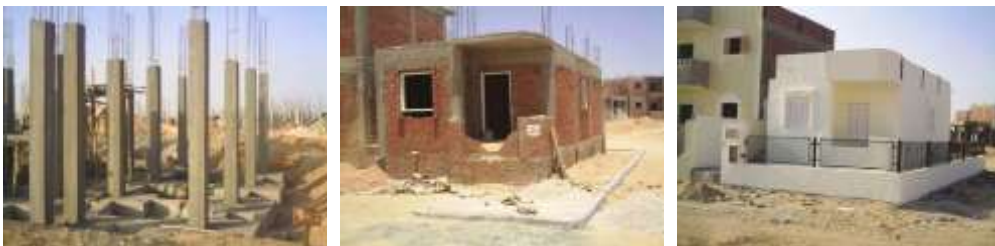
Figure 38: implementation Phases (foundation/columns & walls& finishes) (Source: Fathy, Building owner, Received 2013)
