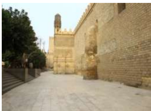
Figure 16: A transitional space in front of Al-Hakim Mosque (Source: Author, 2012)
