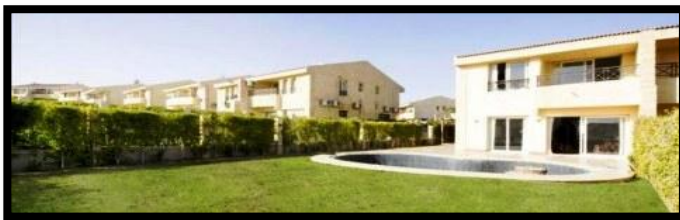
Figure (6.9): View of the walls separating between corresponding villas- Source: www.nileestate.com
