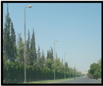
Figure (6.13):View of the street showing the light fixtures installed as a part of street treatments-Source: Author
