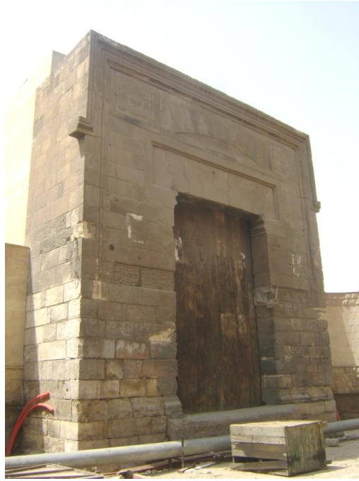
Figure 3.5 The remaining entrance of Wikālat Qawsūn.
