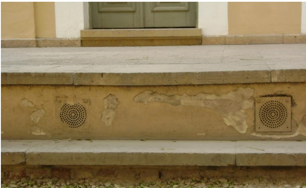
Figure 3.17 Ventilation openings for foundations of Darb Shoghlan school.
