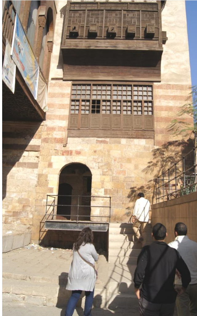
Figure 3.11 Modern steel handrail and entree floor slab implementations in Bait ar-Razzāz, in ad-Darb al-Aḥmar.
