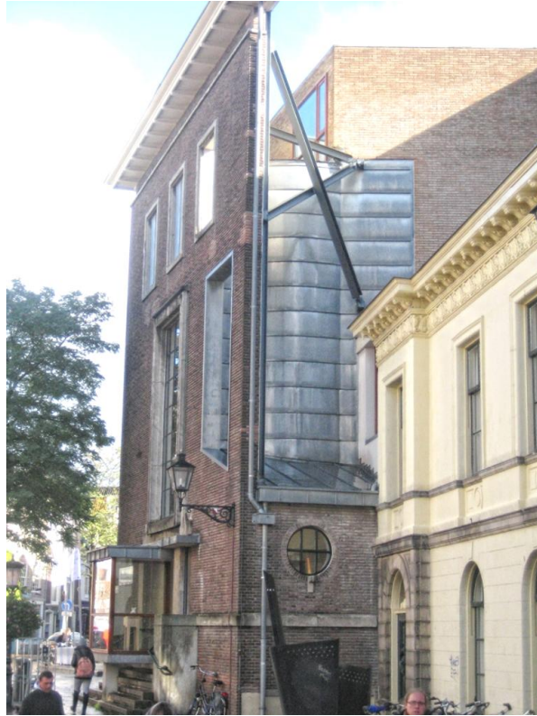
Figure 3.3 Northern façade retention of the City Hall of Utrecht.
