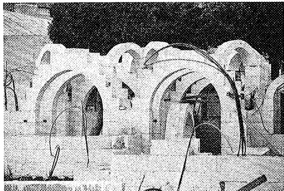
Figure 9: The base of three domes built according to the model.
