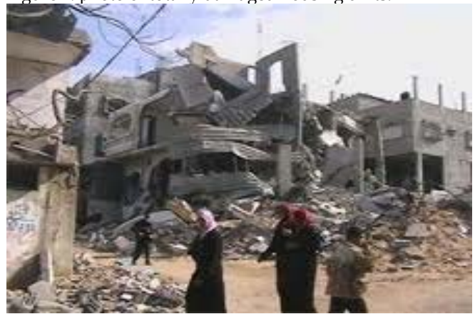
Figure 3: photo of collapse of the building.
