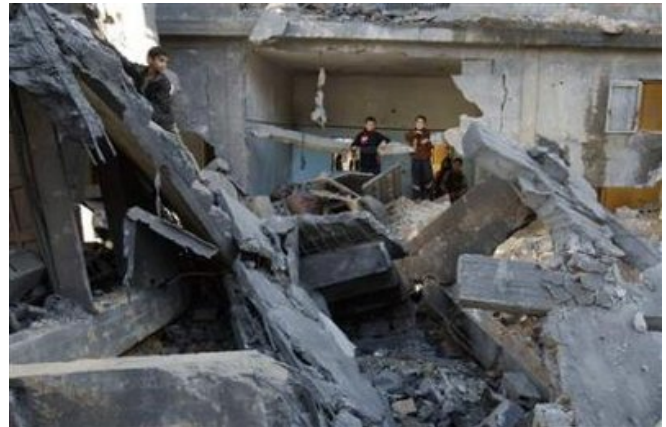
Figure 2: photo of totally damaged housing units.
